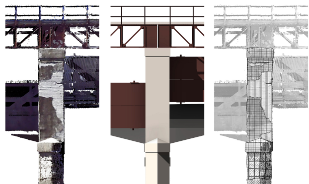
Figure 8. State of deterioration of a pillar (orthophotos, BIM Model and deterioration)
