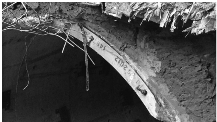
Fig. 4. View of the hardened grout as can be seen in the enlargement for a station. It is possible to observe how the mix fills completely the void annulus (photo Mapei's archive).
