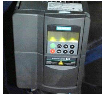
Figure A.11: Fan Control-Unit.
