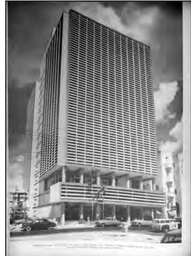
Retiro Odontológico building. Arquitectura , No. 282, January 1957, p.22-30
