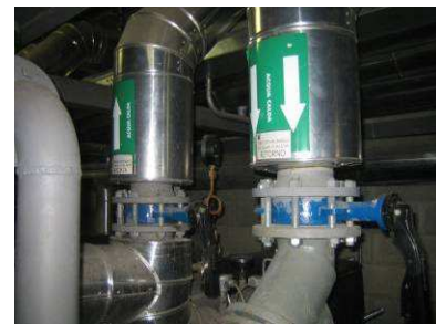
Figure – District heating connection
