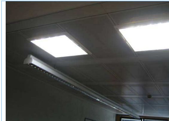
Details of skylights and solar tubes
