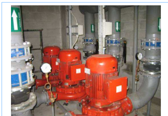
Figure – heat rejection circuit pumping system
