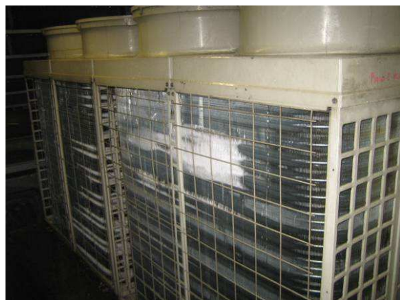
Ice formation on the external units
