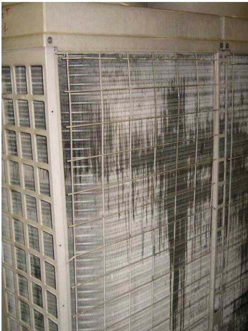
Ice formation on the external units
