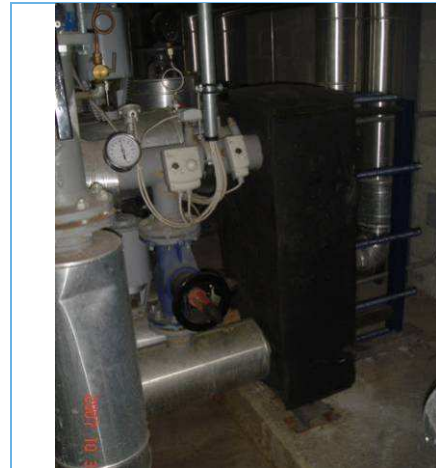
Figure – Heat exchanger
