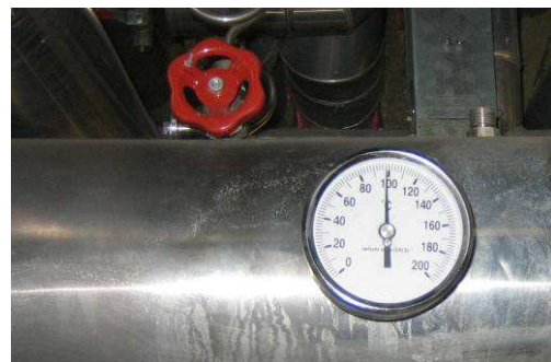
Figure – Temperature of district heating network inlet
