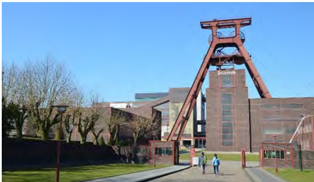
Figure 3-11 Schupp and Kremmer’s pithead buildings and headgear at Shaft 12, Zeche Zollverein, Essen-Katernberg, Germany, representing the past image of Ruhr coal and attracting visitors. (Photo: by author)
