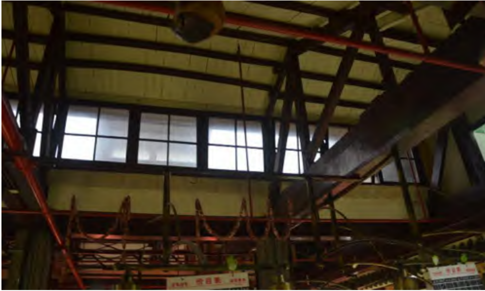
Figure 5-7 Taikang Vegetable Market had successfully moved in the abandoned factories in 1990s (Source: by author)
