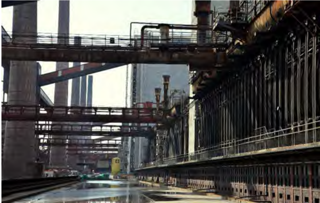
Figure 3-12 Coking plant and the pool(used for ice-skating rink in winter ) in Zollverein, Essen-Katernberg ,Germany. (Photo: by author)
