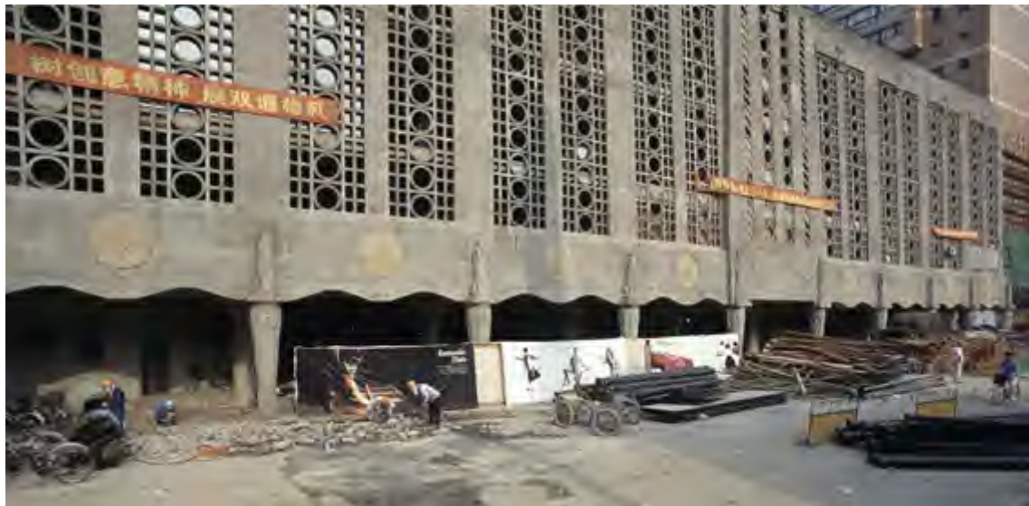
Figure 4-31 The construction site of the restoration project, 2007 (Source: http://forum.xitek.com/forum-viewthread-action-printable-tid-390839.html )
