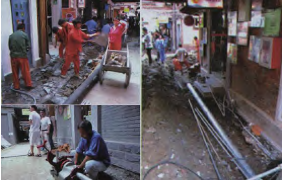
Figure 5-28 The construction site 2008 (Source: KE Xiongbin and others, “The Protection of Characteristic Streets in Modern City: A Case Study of Shanghai Tianzifang,” HUAZHONG ARCHITECTURE, 2011, 184–188.)
