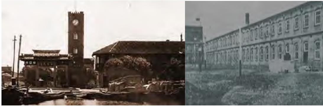
Figure 1-9 The Ta Sheng Cotton Mill in Nantong was built by Zhang Jian, one of the leaders of private enterprise at the end of 19th century. As a typical factory the development of national modern industry in China, it has been appointed as Major Sites Protected for their Historical and Cultural Value at the National Level in 2006, including the original bell tower, workshops designed by American architect, official and residential buildings. Now the whole area is being transformed in to a creative park. (Source: http://www.ntda.gov.cn )
