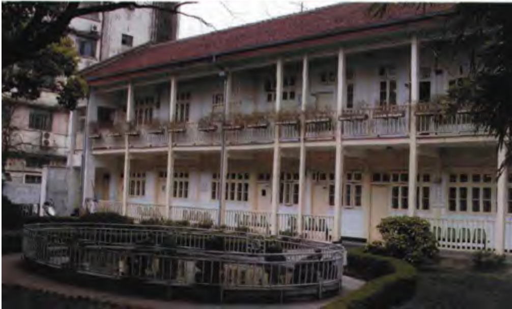
Figure 2-28 The protected office building in Jiangnan Shipyard (Source: Yun-qi, CHEN, YIN Jian-ping, and LIU He, “Let the ‘Jiangnan Culture’ Stay beside the Huangpu River:Preliminary Study of the Conservation and Rehabilitation of Jiangnan Shipyard,” TIME ARCHITECTURE, 02 (2006), 67–71)
