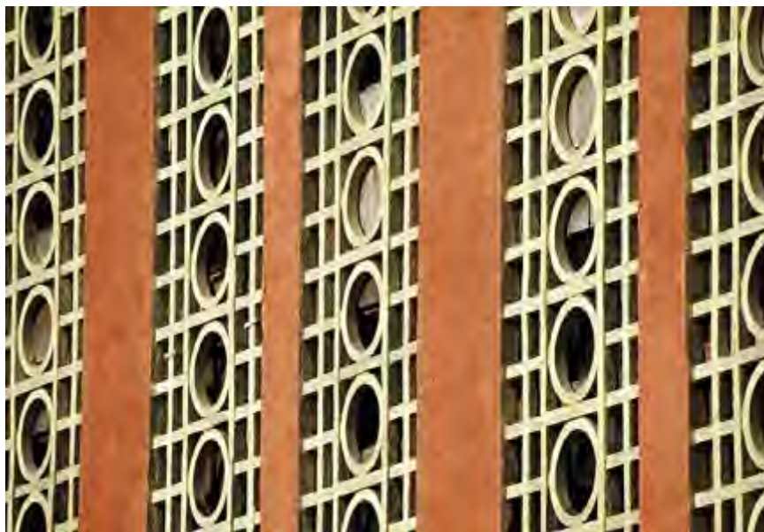
Figure 4-29 The external wall coated a layer of pink, 1# Building, before the restoration (Source: http://forum.xitek.com/forum-viewthread-action-printable-tid-390839.html )
