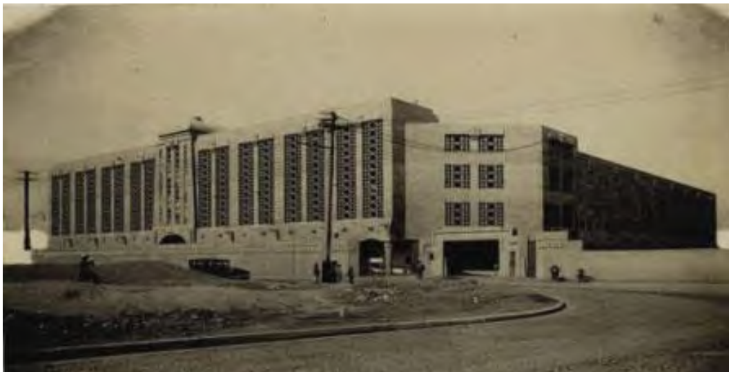
Figure 4-4 Shanghai Municipal Abattoir in 1937 (Source: Shanghai Municipal Archives.)
