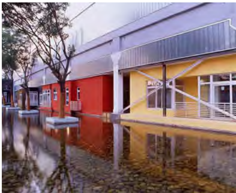
Figure 2-34 Ocean Art Center, renovation by architect Yung Ho Chang, Beijing (Source: http://www.oceansky.net.cn/Article_end.asp?10200.shtml )
