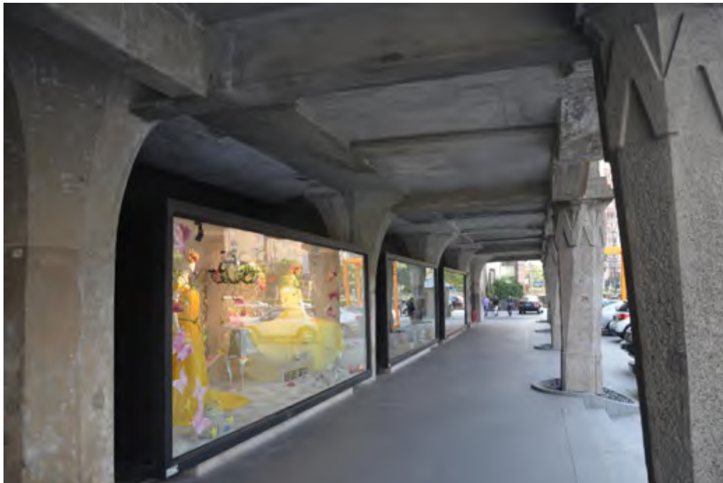
Figure 4-33 Ornamental designed pillars and showcase below the arcade at the side of west facade, 1933 Old Millfun after restoration (Photo: by author)
