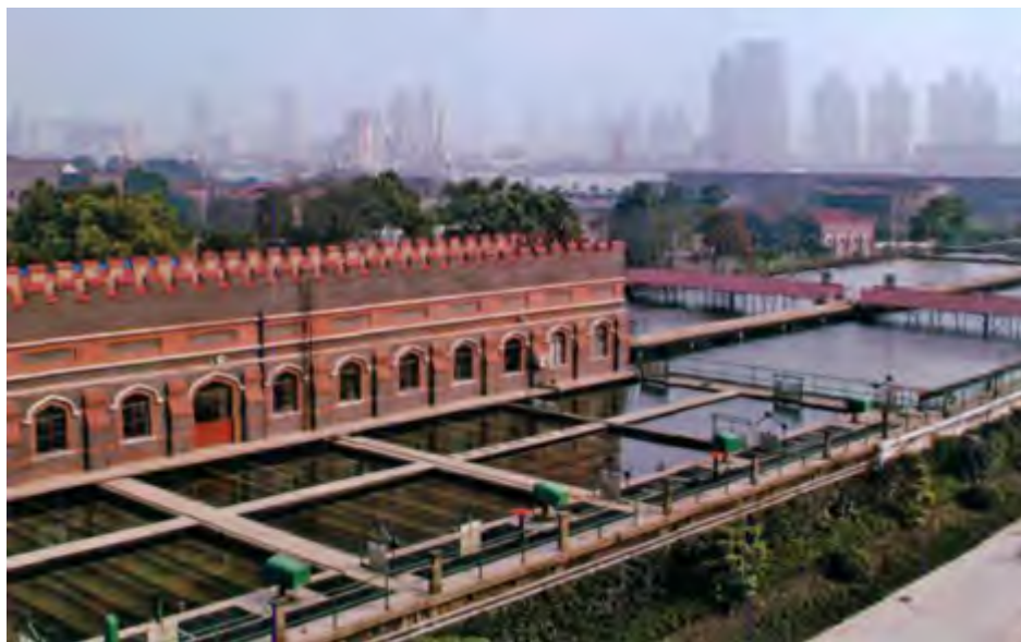
Figure 2-5 Yangshupu Water Plant, listed as Major Sites Protected for their Historical and Cultural Value at the National Level. It changes a shutdown workshop into Shanghai Tap Water Pavilion and other parts continue the previous function (Source: Zhang, Song, and Li, Yuxin, “Exploring the Strategy of Integral Conservation Planning for Yangshupu District in Shanghai,” ARCITECTURAL JOURNAL, 2012, 18–23)
