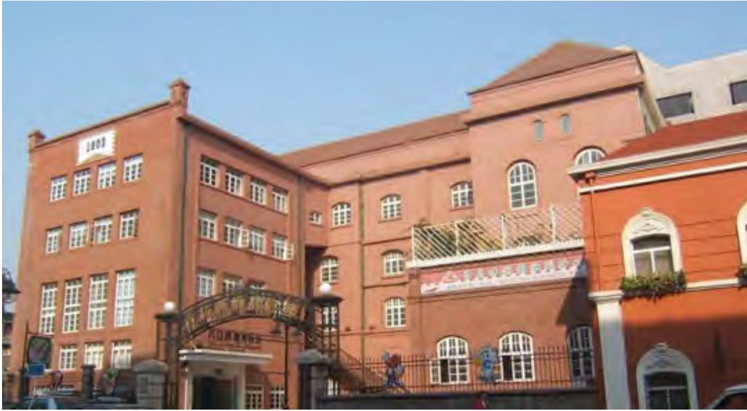
Figure 1-11 Tsingtao (now Qingdao) Brewery is China's first beer factory that built by German beer company in 1903. The early buildings of the Tsingtao Brewery have been appointed as Major Sites Protected for their Historical and Cultural Value at the National Level in 2006. Now this Jugendstil style, red brick building is re-used as Qingdao Brewery museum to present the production of beers together with other factory buildings in use. (Source: http://www.tsingtaomuseum.com )
