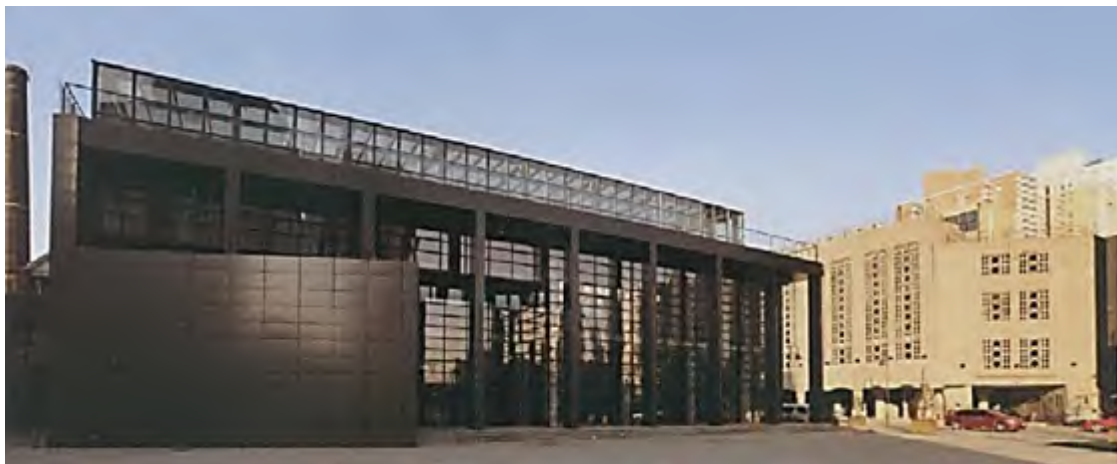
Figure 4-26 The 4# building after restoration, 1933 Old Millfun (Source: Chongxin ZHAO, “Reconstructing of 1933 Old Mill,” Architectural Creation, 2008, 50–56)
