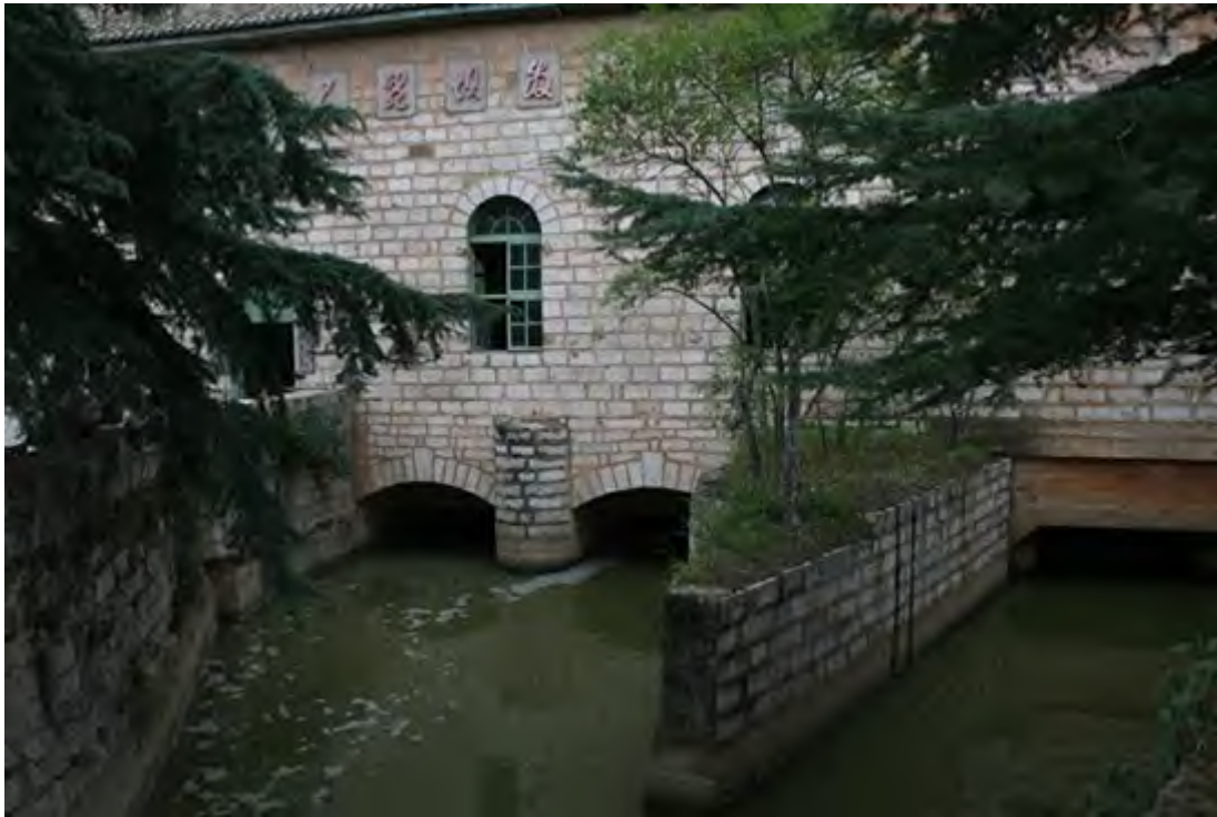
Figure 1-13 Shilongba hydropower, built by Chinese enterprisers in the year of 1910 and equipped two Siemens motors, is the first hydropower project in China. It has been appointed as Major Sites Protected for their Historical and Cultural Value at the National Level in 2006, including the dam, offices, residential buildings and the machines. Now some buildings are renovated as part of a hydropower museum. (Source: http://yn.zwbk.org/lemma/3801 )
