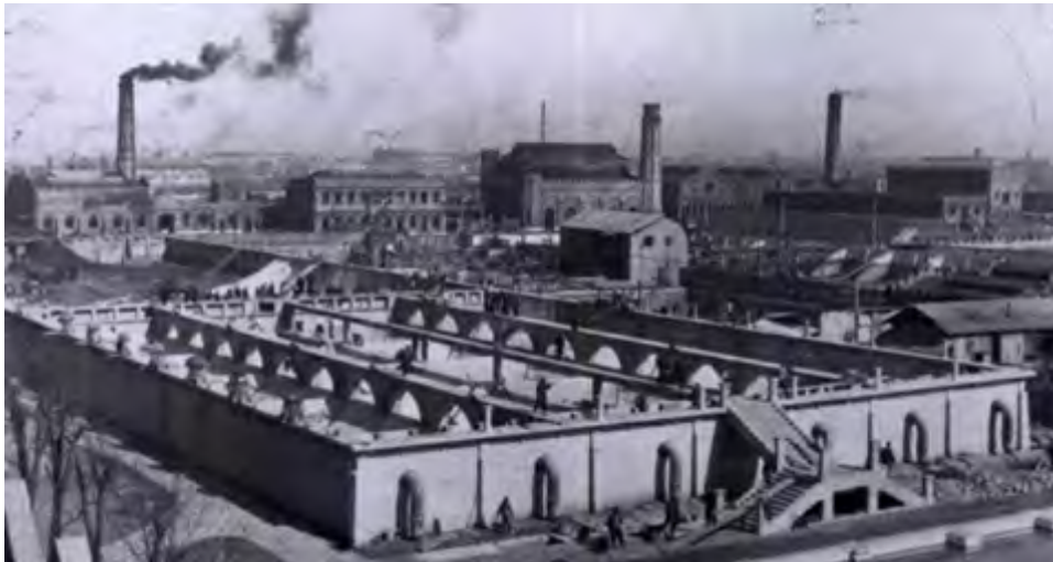
Figure 2-4 the original appearance of Yangshupu Water Plant at the end of 19 th century(Source: Zhang, Song, and Li, Yuxin, “Exploring the Strategy of Integral Conservation Planning for Yangshupu District in Shanghai,” ARCITECTURAL JOURNAL, 2012, 18–23)
