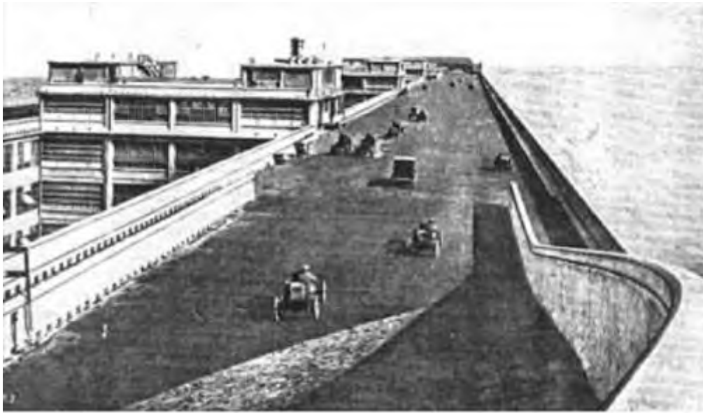
Figure 3-1 The Fiat Lingotto roof with its testing track in action, as published by Le Corbusier in Vers une architecture to illustrate the fusion of engineering, speed and clean structure (Source: Gillian Darley, Factory (Hong Kong: Reaktion Books, 2003), p. 224.)
