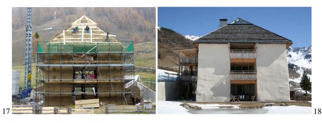
The experience of house Fliri showed even better structural performances (Fig. 17-18): 1 linear metre of straw-bale wall, plastered on both sides, can carry 1+3+1 tonnes instead of 1+0.2+1 as according to the American construction method and structural model. Braun thinks the major static issue is not maximum admittable load, but creep control, so to keep the floors horizontal.
