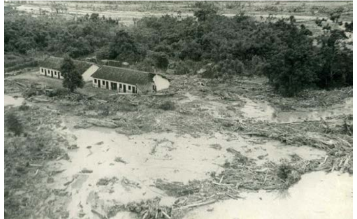
Figure 5. Destruction in the dock area and Packing House of English Farm after the debris flow of March 1967.
