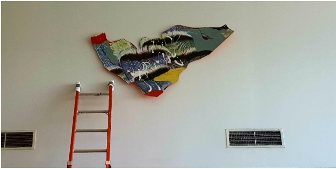
A test piece was hung to determine installation method and stability.
