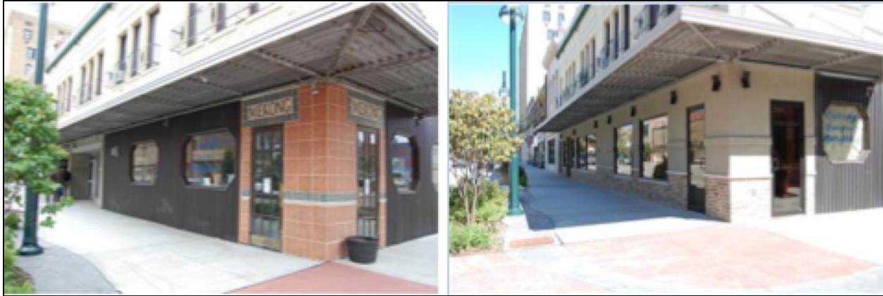
Figure 9: Moline façade improvement
