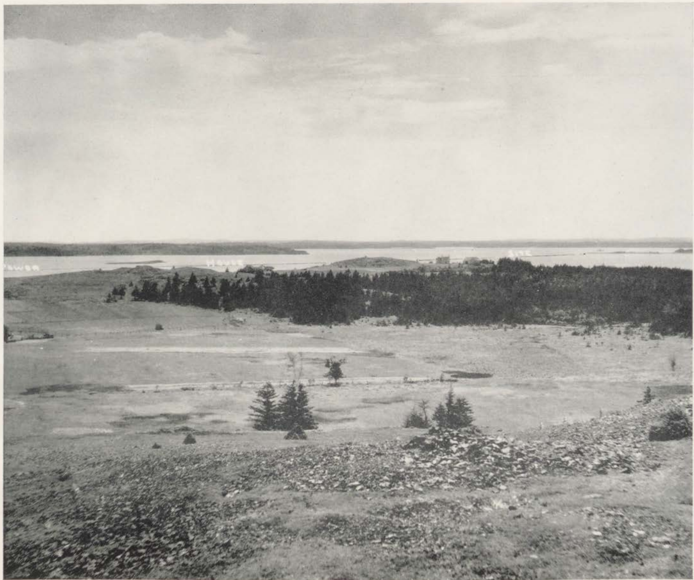
Power House Site, Eastport
