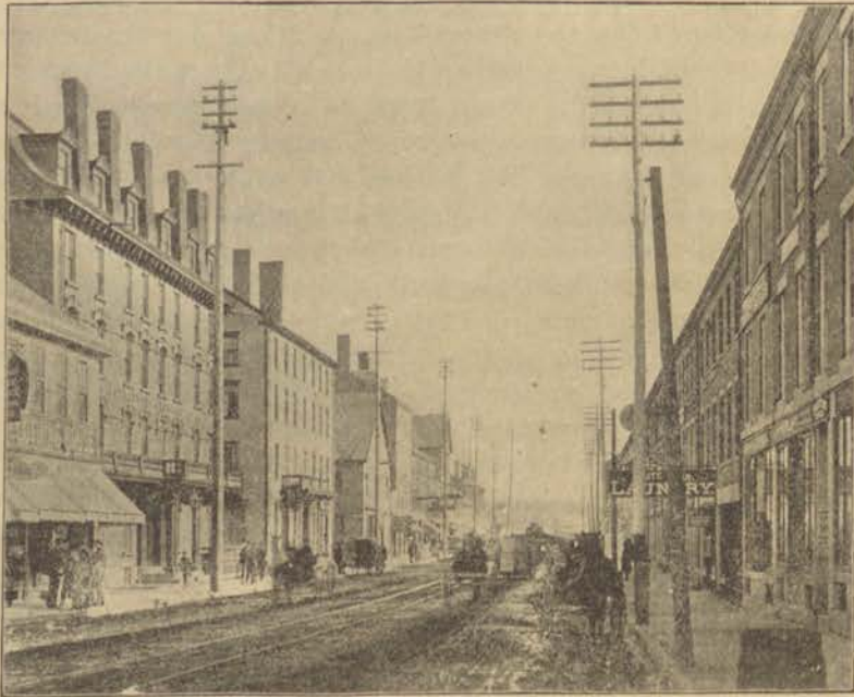
EXCHANGE STREET, LOOKING TOWARD RIVER.
