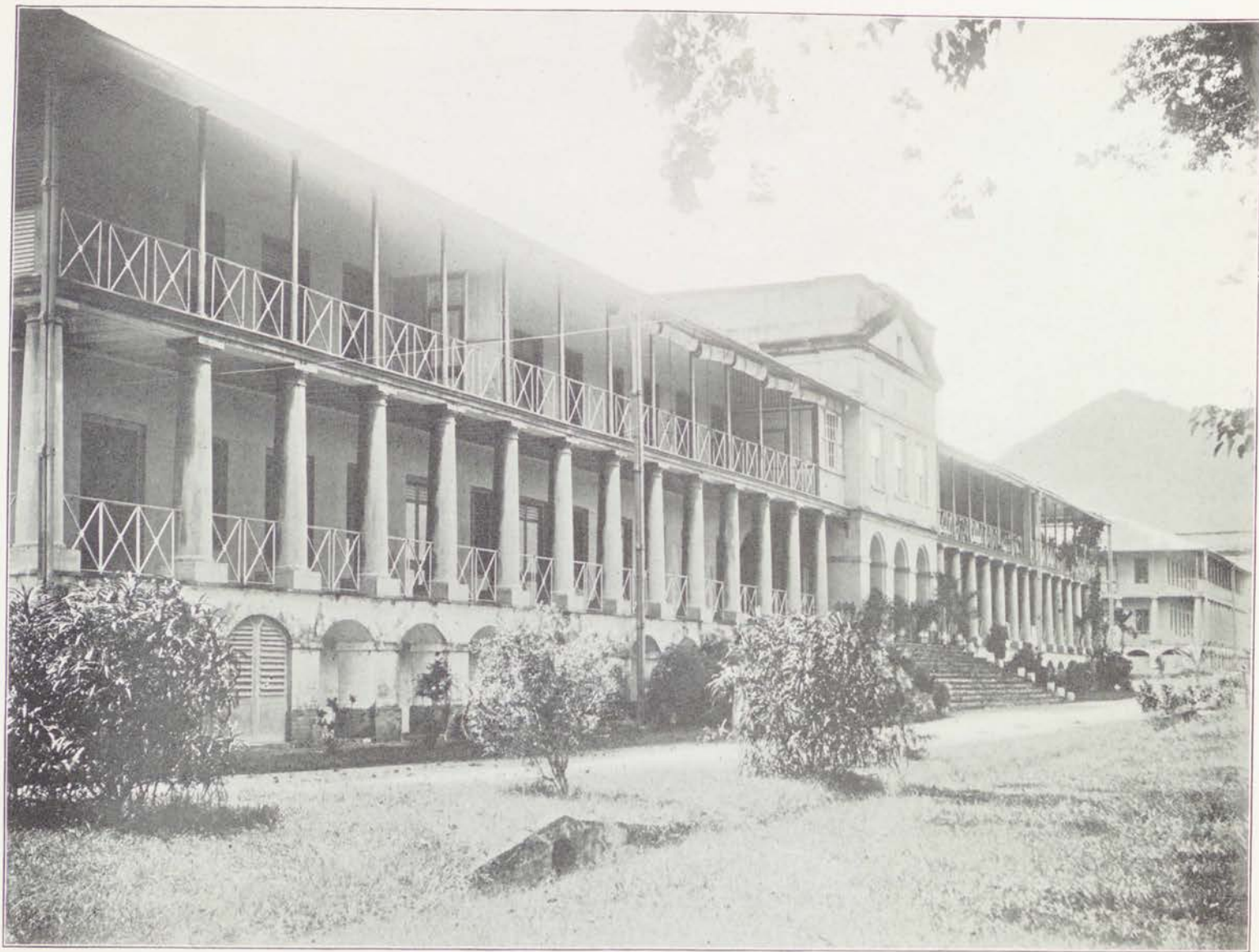
ST. JAMES' BARRACKS
