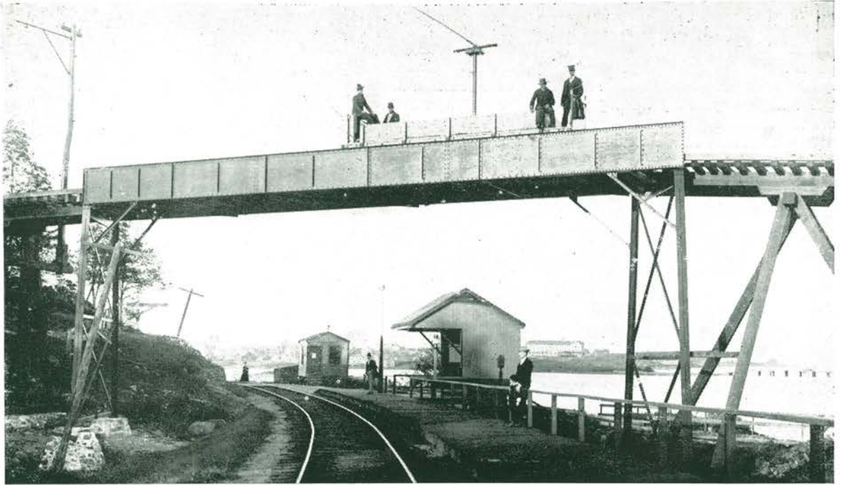
TRESTLE of the Portsmouth, Kittery & York Street Railway over the York Harbor & Beach Railroad at Seabury in York, Maine. Car on trestle is single truck flat "B." —Collection of Howard T. Moulton.
