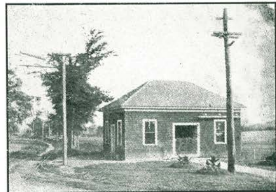
A NEAT SUB-STATION AND WAITING ROOM AT YORK CORNER, MAINE
