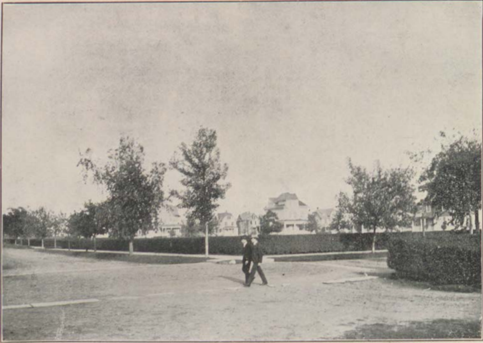
CORNER 12TH AVE. AND 49TH STREET, BOROUGH PARK, NEW YORK CITY, IN 1904
