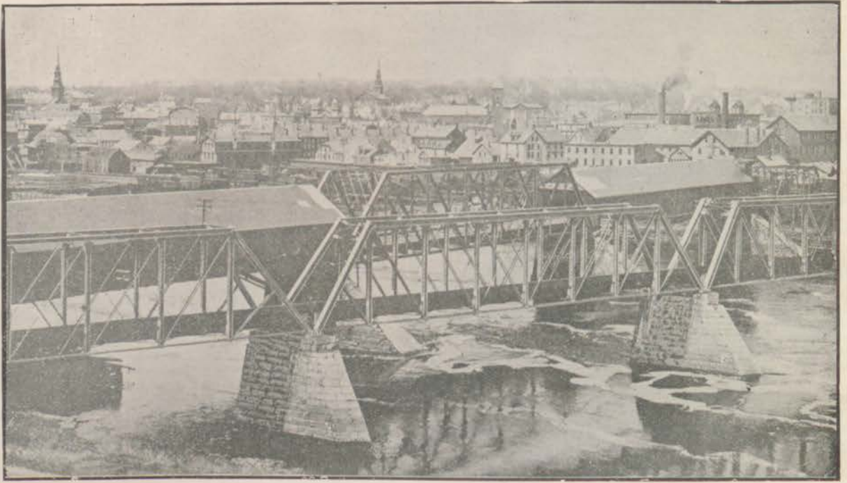
BANGOR FROM RAILROAD BRIDGE.
