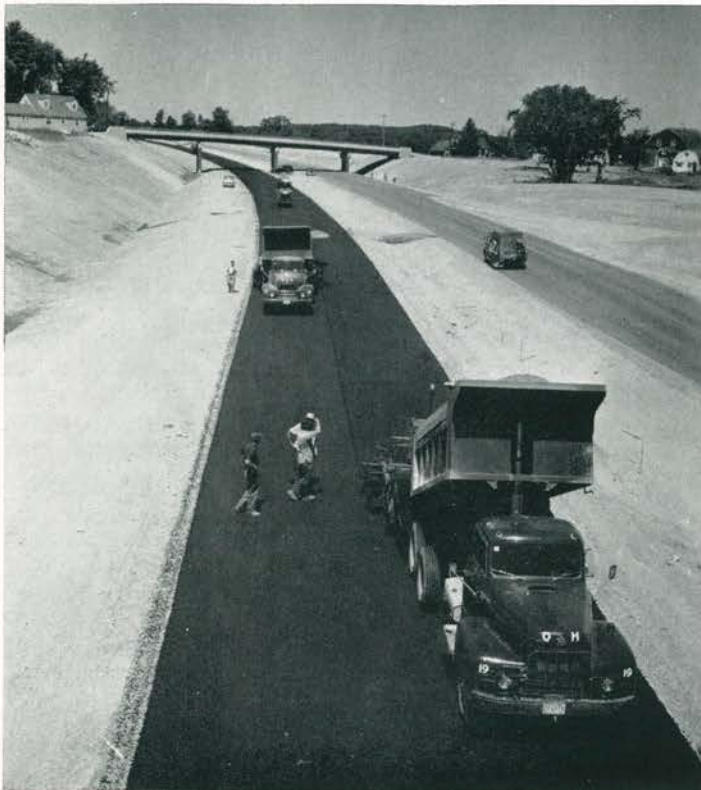
before final paving
