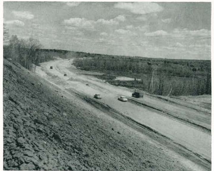
must be laid . . .
