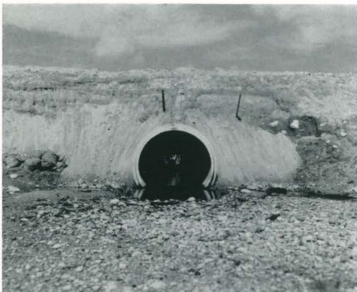
of big drainage pipe . . .
