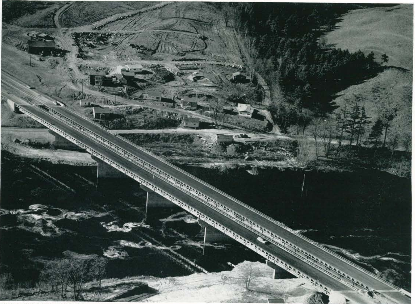
THE LONGEST BRIDGE of the 91 bridges on the Maine Turnpike extension is the 846-foot structure over the Androscoggin River at Lewiston. Built by W. H. Hinman, Inc., North Anson, Maine.
