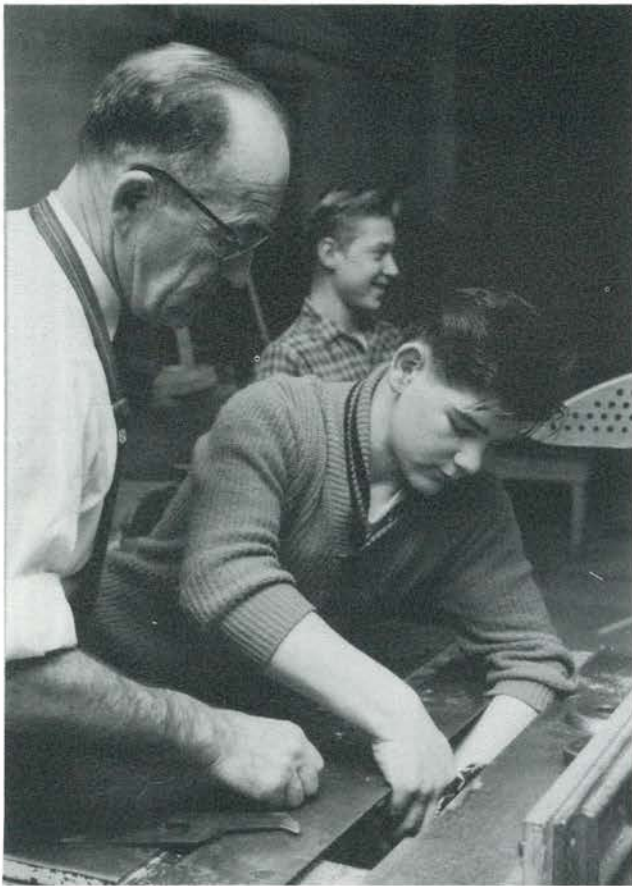
Under Mr. Landerkin's guidance, Gary Hachey sets up a dado head.
