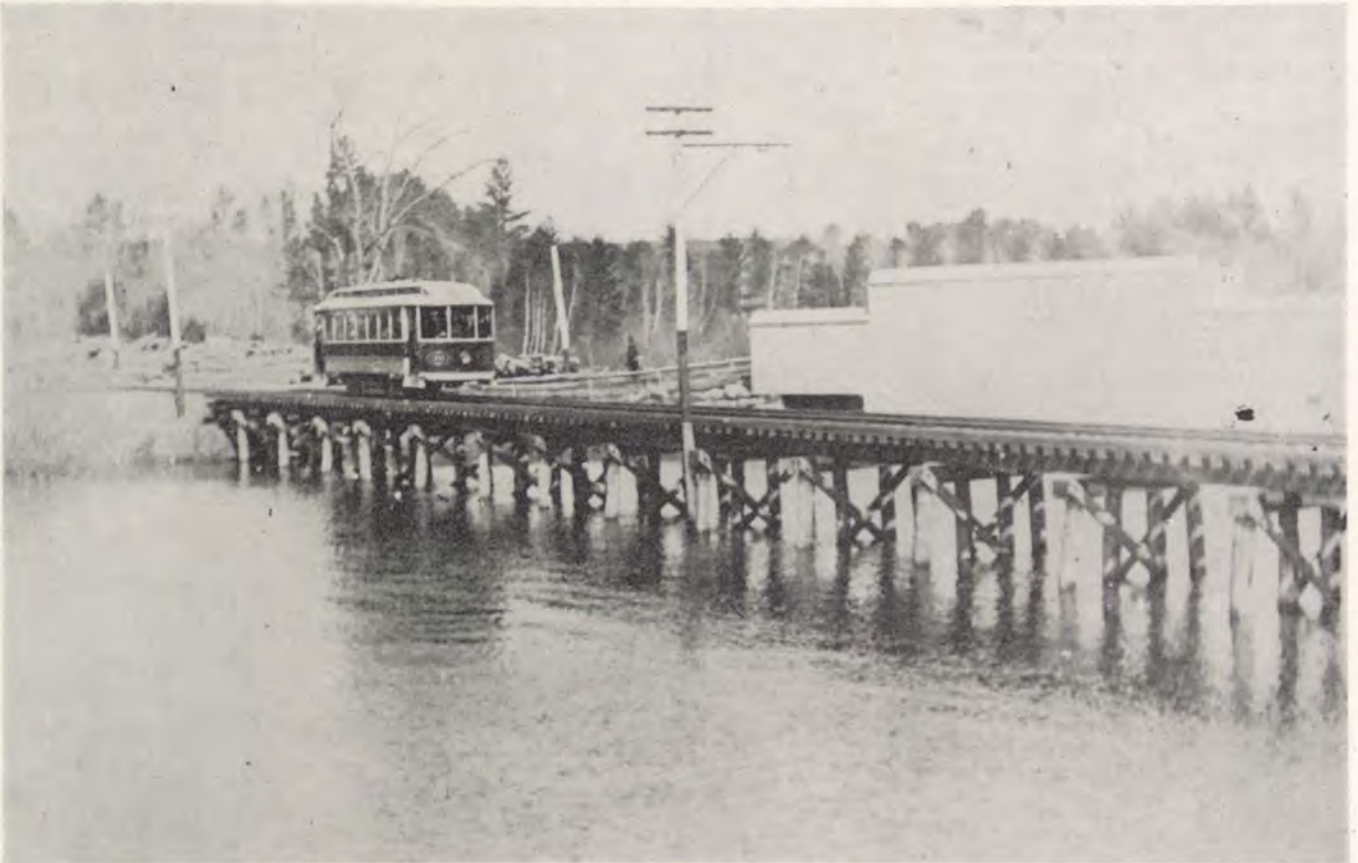
NEW MEADOWS RIVER pile trestle, showing car No. 38, one of the Briggs 20-foot closed cars purchased for the Lewiston-Bath service in 1898 by the Lewiston, Brunswick & Bath Street Railway Co. —[Lancaster Collection.
