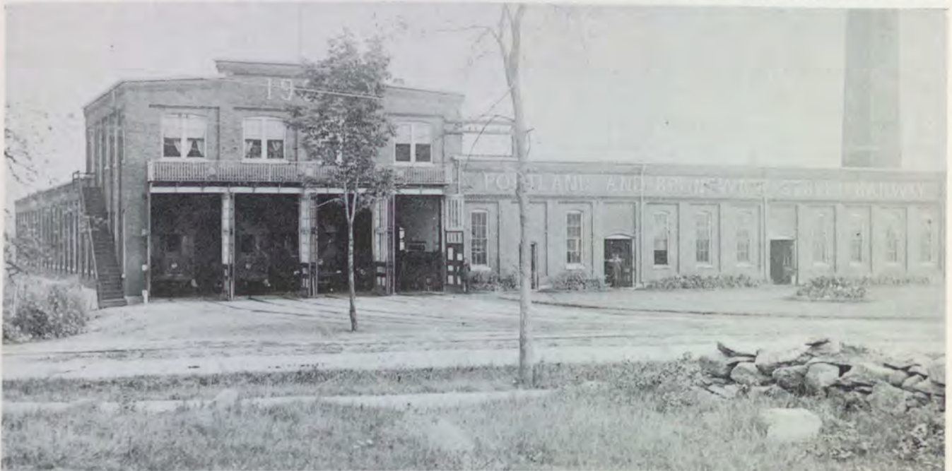
FREEPORT carbarn and power station of the Portland & Brunswick is shown about 1906. —[Photo by Don Welch.
