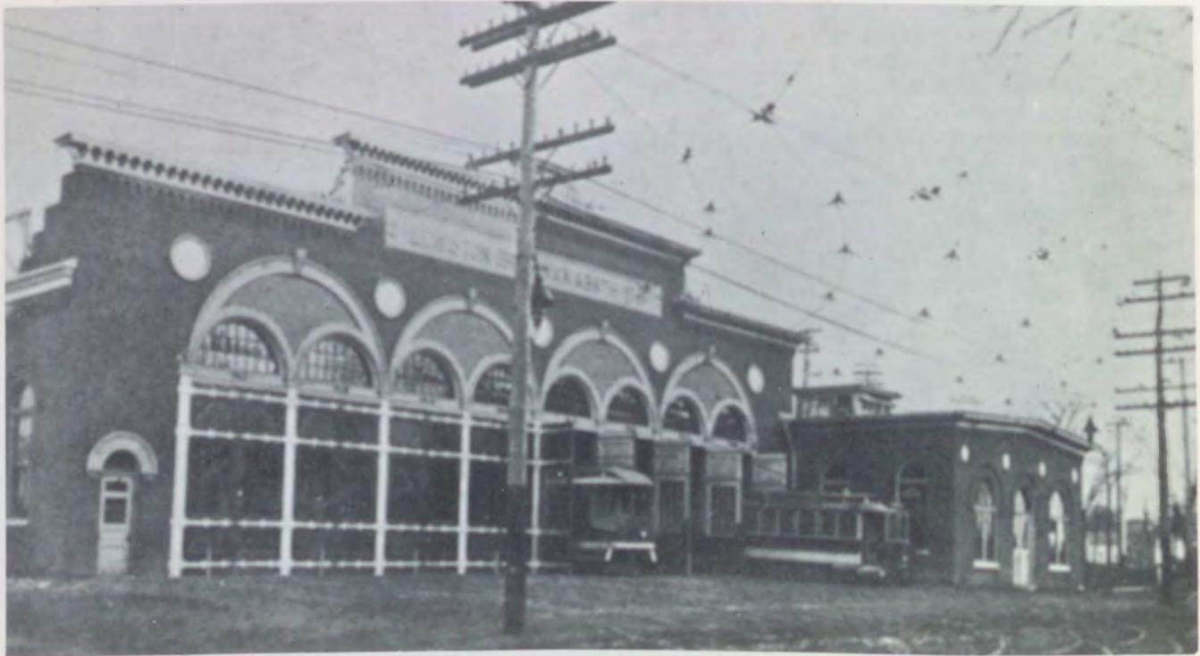
FIRST CARHOUSE at Lewiston, as constructed in 1899. The building was destroyed by fire on December 19, 1903, and was replaced by a new carhouse which continues to serve (1966) as a bus garage. —[Cummings Collection.
