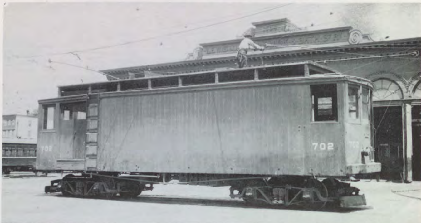
LINE CAR ON THE JOB — No. 702 is shown in front of the Lewiston carbarn on Lisbon Street while lineman makes some minor repairs on the overhead trolley wire. —[Photograph taken on June 30, 1937, by Roger Borrup.
