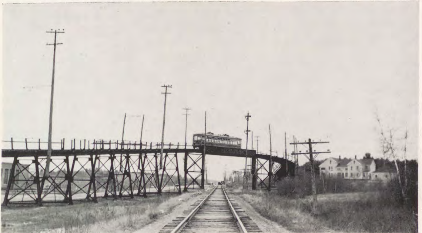
CROOKED BRIDGE over the Maine Central Railroad in South Lewiston on the Lewiston-Lisbon Falls line, as it looked when the lightweight cars ran in Sunday service between 1937 and 1941. Note that high tension wires were carried on same pole line as the trolley wires. —[From a photograph taken by Gerald F. Cunningham.
