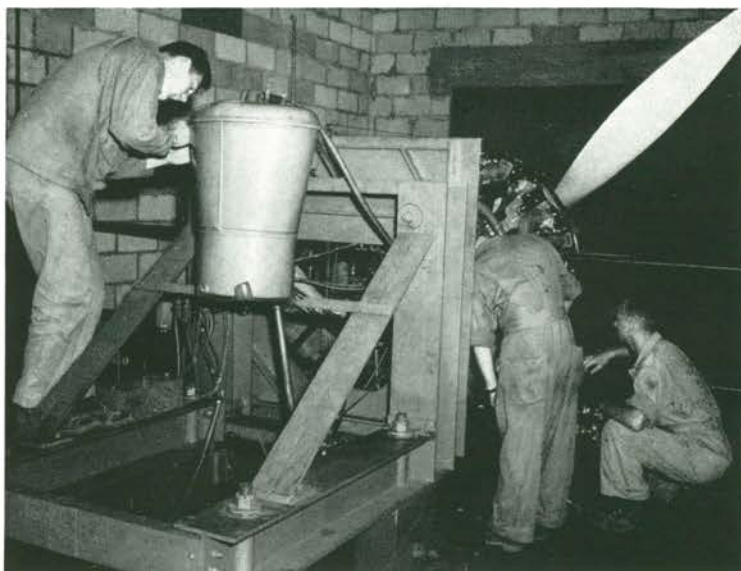
Pre-flight Inspection on R-2600 Engine.
