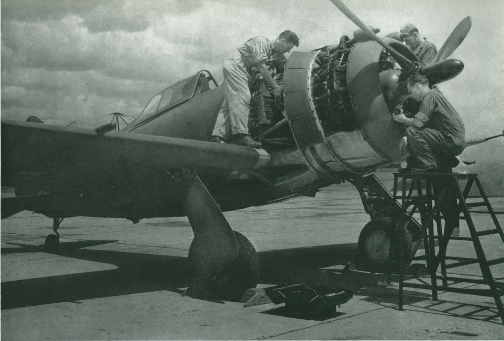
50-HOUR INSPECTION OF GENERATOR AND PROPELLER BRUSH LENGTH ON P-43 PLANE
