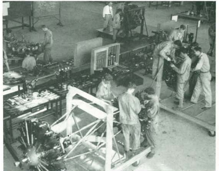
Part of the Engine Change Branch Work Room.
