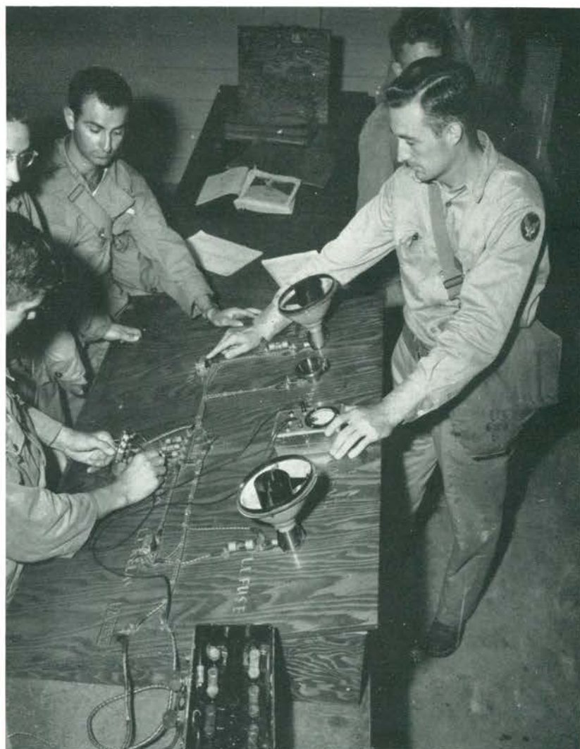
Explaining Electrical Blueprint.
