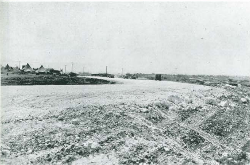
Shown here are three views of Route No. 6 constructed by the 145th from Hiza up the west side of the island along the beaches for about five miles. One of the island's heaviest traveled roads during the Okinawa campaign, this artery was built extra wide and heavily coraled.
