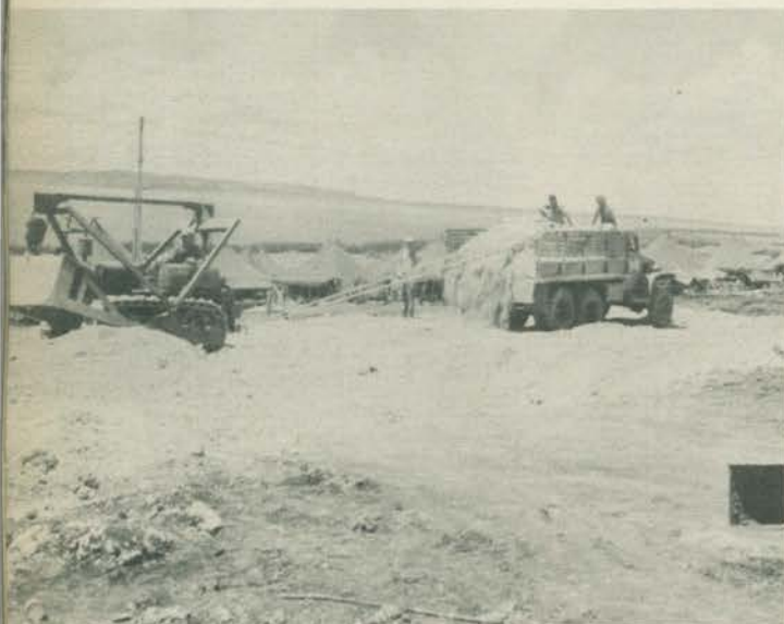
Road construction in September of 1944
