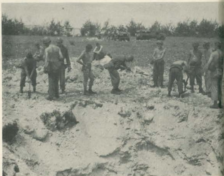
Beginning of latrine construction
