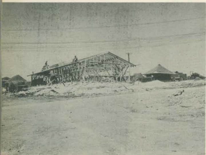
Mess hall construction—October 1944
