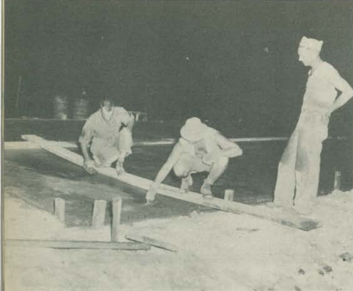
Construction work went on all night in early days.
