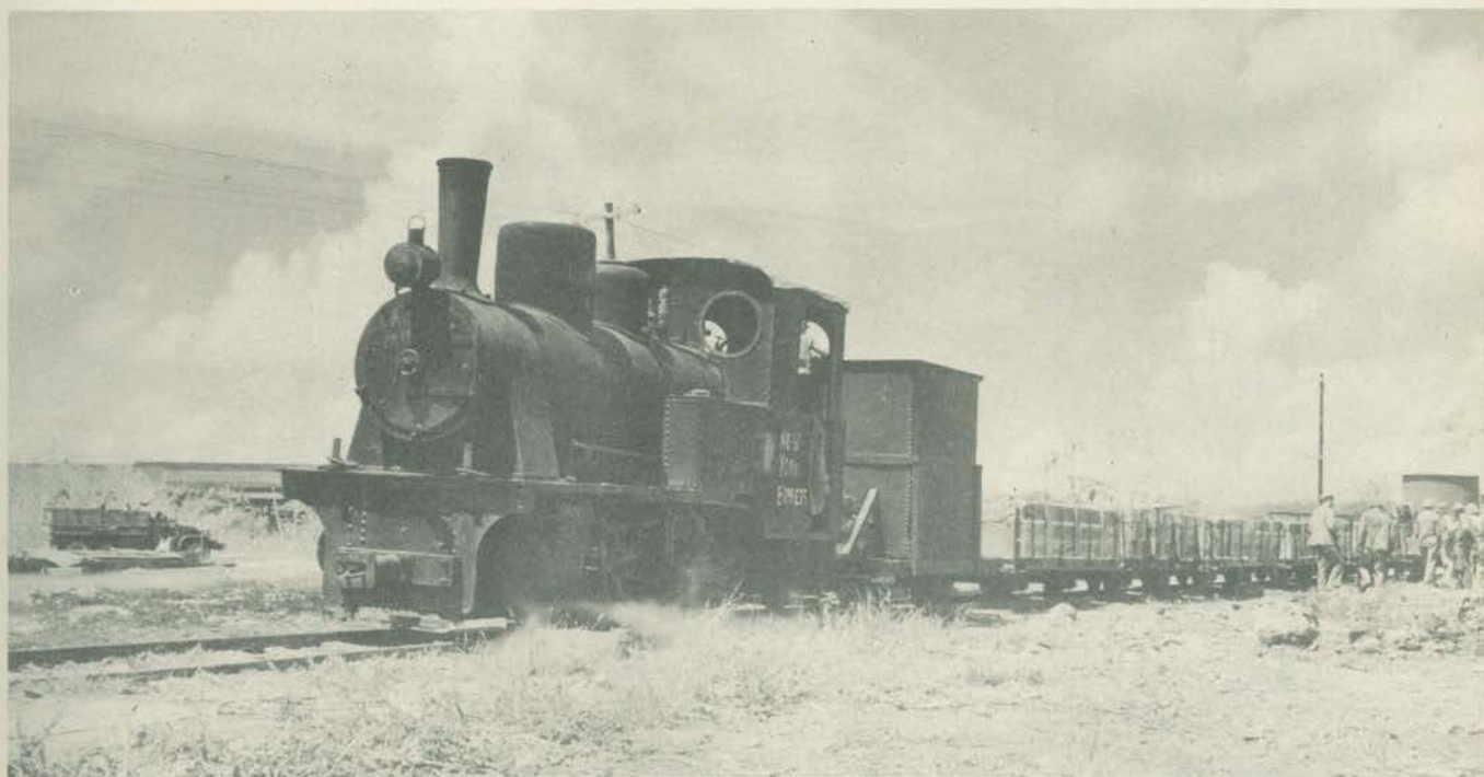
Captured Jap railroad engine and cars being used by the Navy Sea Bees to haul material for airfield repair and construction
