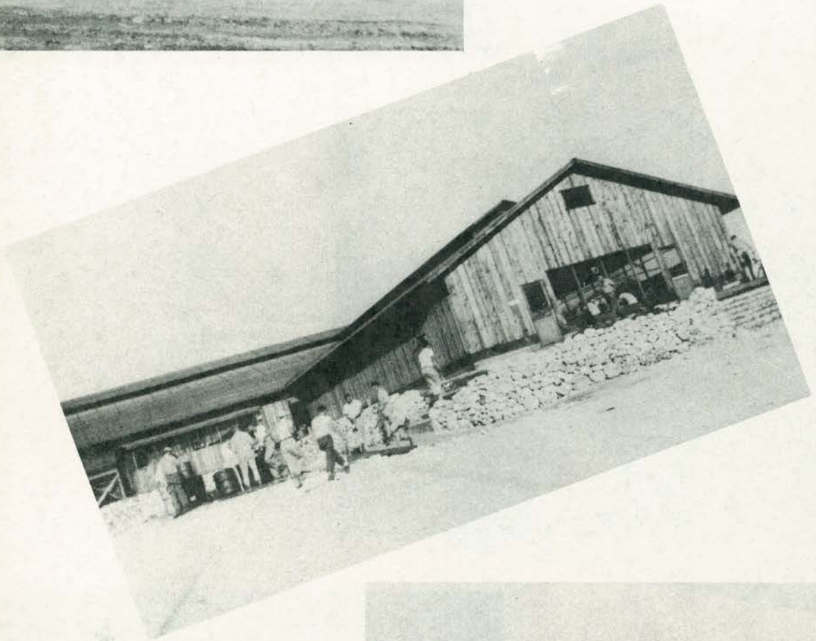
Mess Halls were completed
