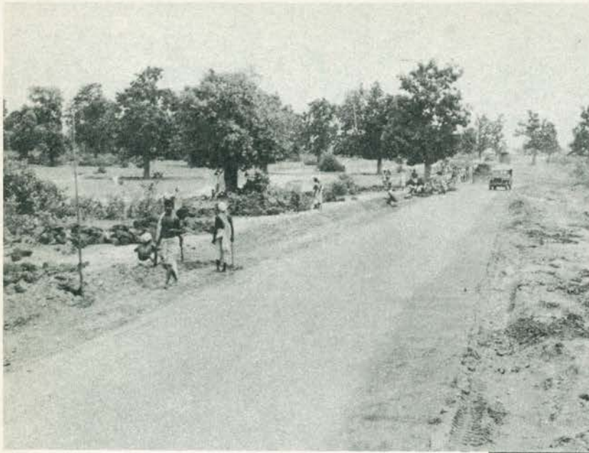
Road Repair Gang (110)
