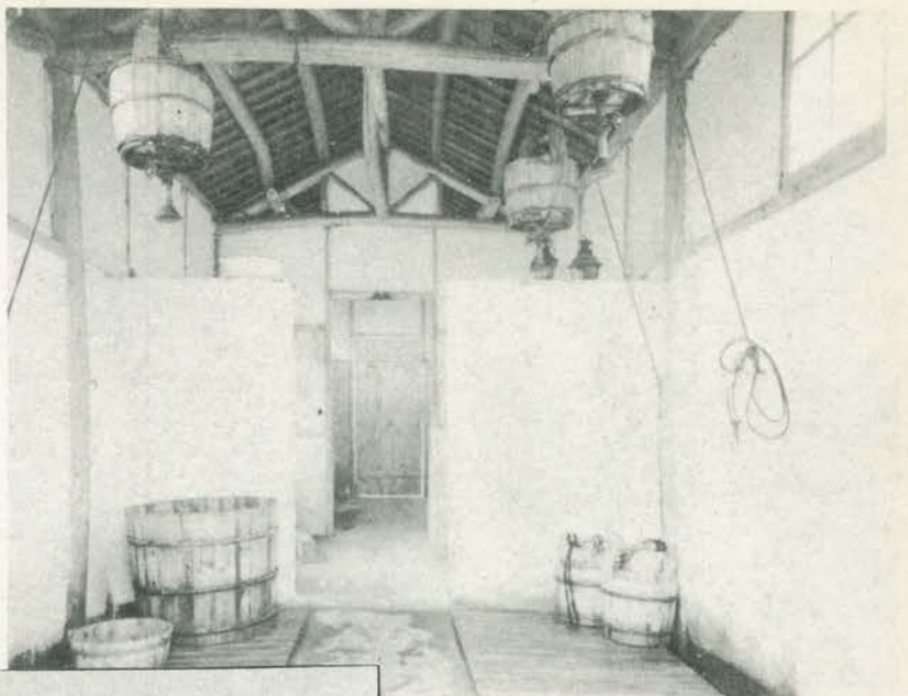
Shower and washroom at Hostel #2
