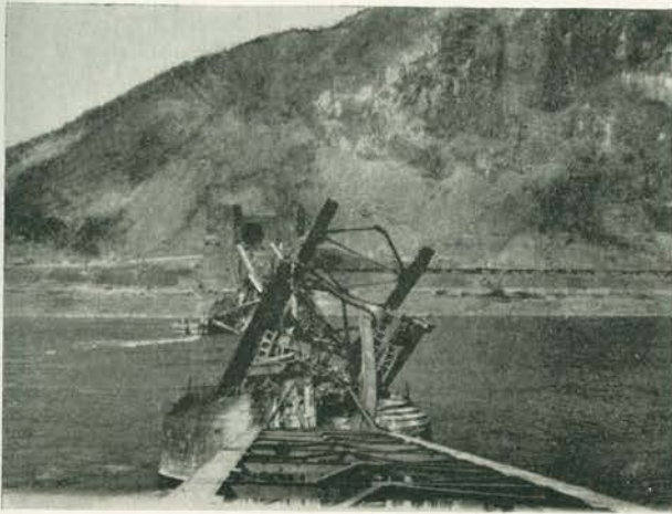
AND LATER — This is the same bridge after incessant shelling caused it to topple into the Rhine.
