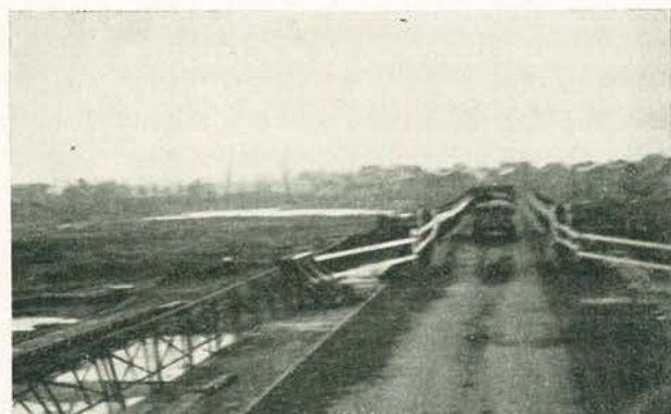
ERFT CANAL CROSSING — Jealous keeps pace with forward elements enroute to Cologne.
