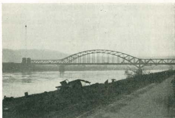
LUENDORF BRIDGE — As it appeared when Jealous crossed the last water barrier in the heart of the Reich.
