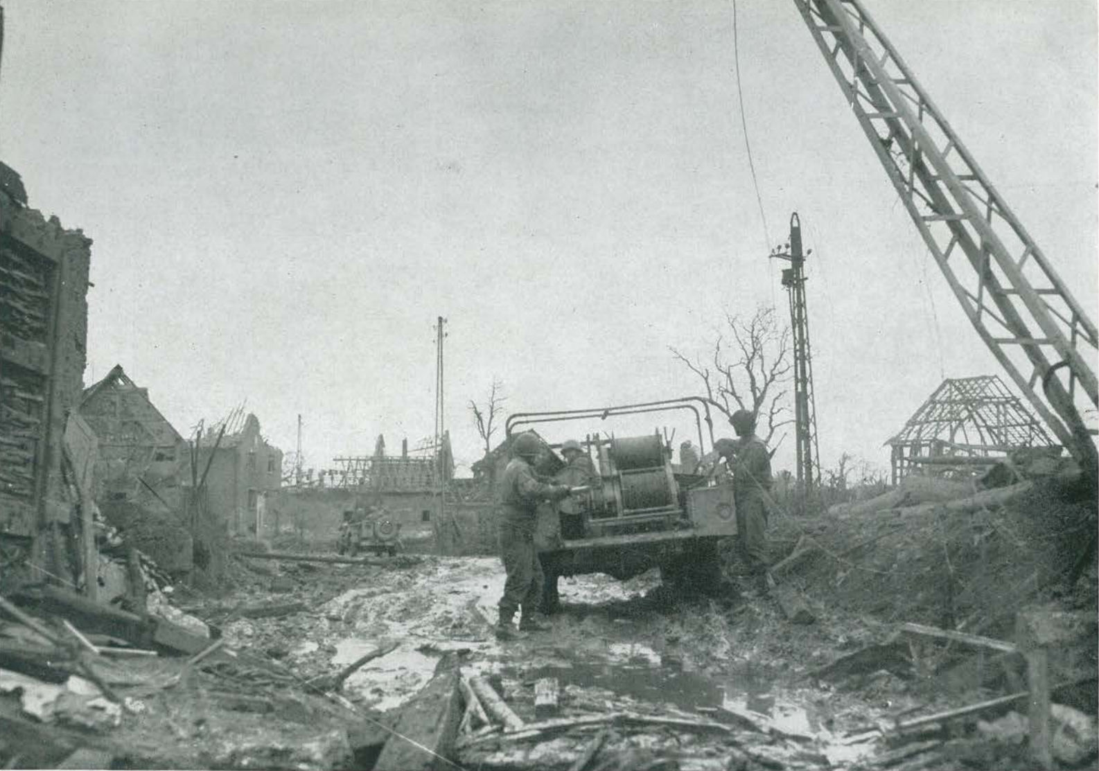
The crew of a forward observation wire team lays wire for a forward observations post in Stockheim, Germany.
