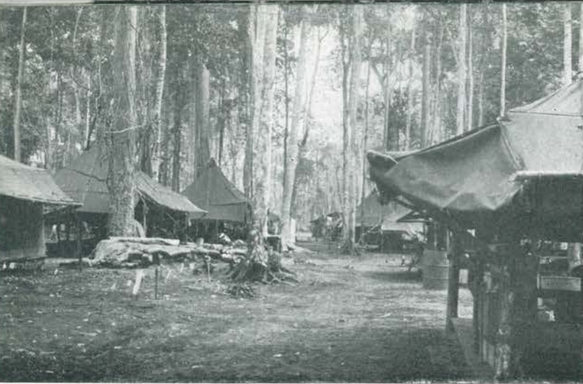
With the jungle cleared, foxholes tidied up, the camp began to look a little better.
