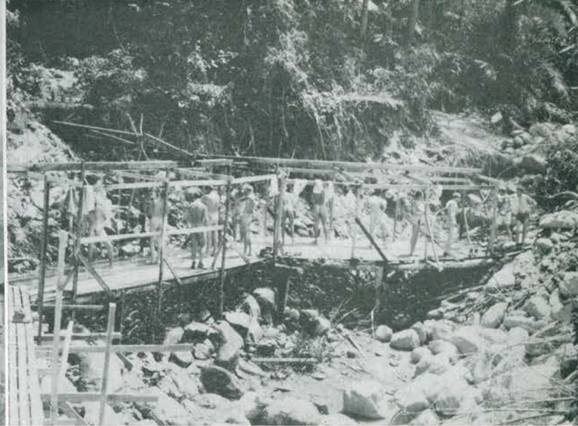
The far-famed Hollandia shower. A waterfall poured down from the left rear, was routed through U-shaped troughs and furnished an abundance of clear COLD water.
