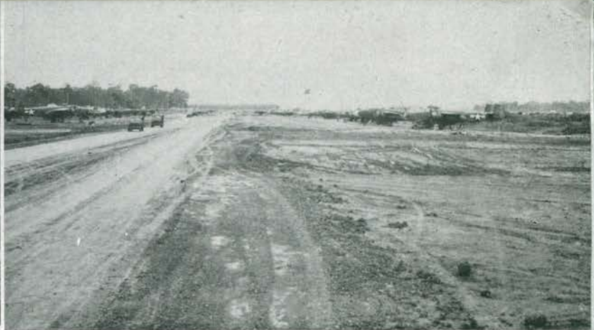
A part of the taxiway and parking area at Palawan. It took weeks of work by the Seabees before things looked like this.
