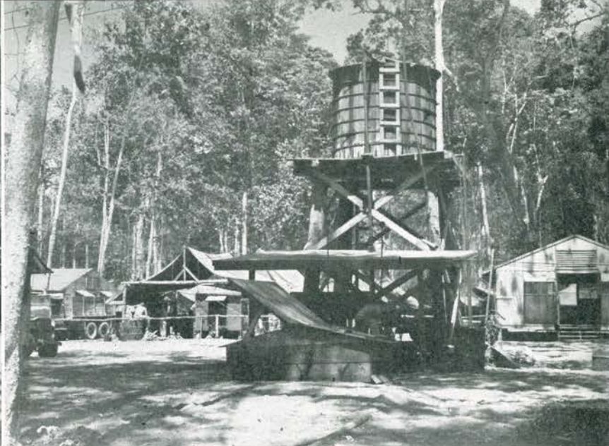
The Group water tower. The water table was seldom below 15 feet, so wells were easy to sink.
