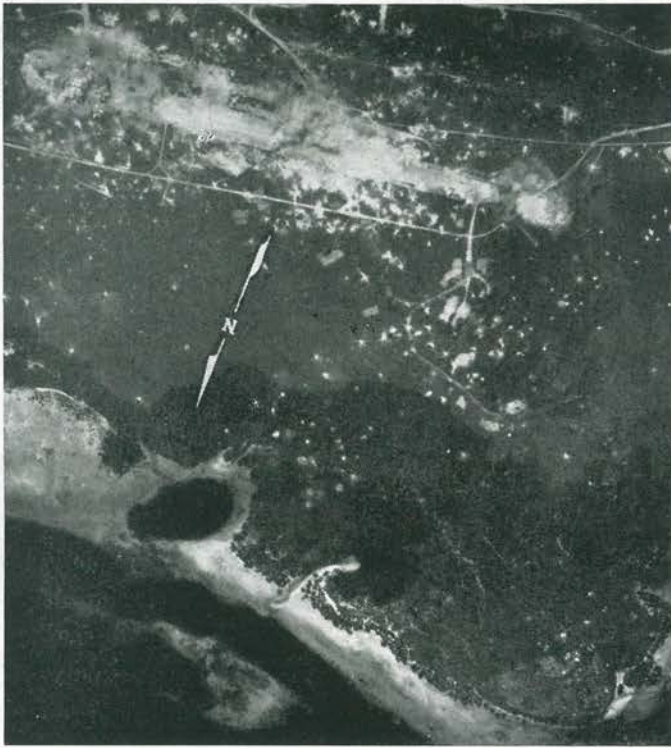
Haroekoe Airdrome, another Jap installation in the Ceram area gets its face changed on December 28, 1944. The strike left it out of operation.
