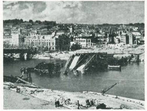
Bombed-out bridge, Rouen, France.
