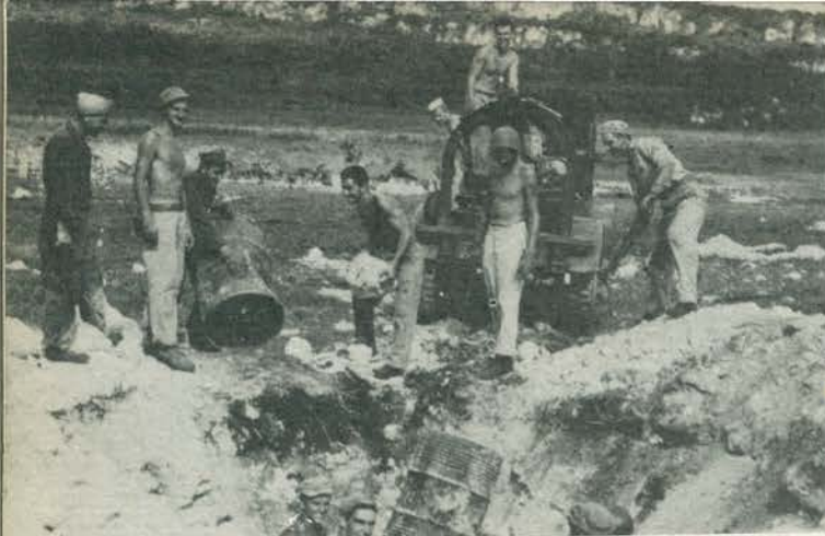
Blasting latrine hole
