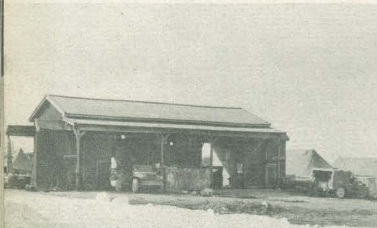
A Jap building on Saipan. Few are still standing.
