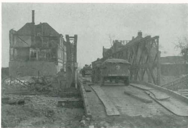
Vehicles of the 79th Infantry Division roll across a newly constructed Bailey bridge spanning the Rhine-Herne Canal near Essen, on 8 April 1945, as the Division continued its drive on Essen.
