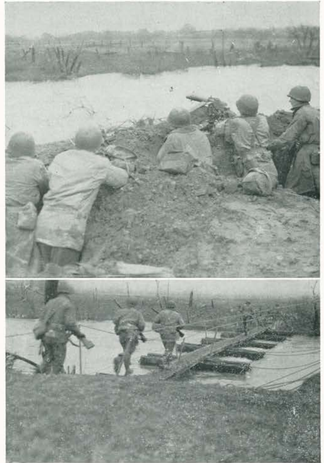
Initial crossings of the Roer River at Hilfarth were made by footbridge. At top, machine-gun crews fire a protective screen as engineers hasten bridging operations. Below, infantrymen of the 35th Infantry Division cross on the completed bridge under enemy fire.
