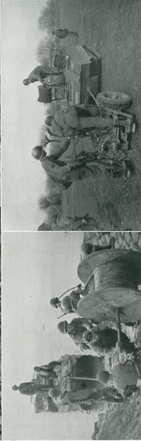
At upper left, a 97th Signal Battalion sign painter gets an OK from his first sergeant marking the location of communications cable across the Rhine River from Borth, Germany. At upper right, a Signal Battalion cableman identifies pairs on a German underground cable used to carry telephone conversations on the XVI Corps front near Borth, Germany. At lower left, linemen roll a reel of submarine cable ashore on the east bank of the Rhine River after the cable had been laid across the river by means of the amphibious vehicle in the background. At lower right, spiral-four cable, commonly used throughout all XVI Corps operations for wire communications, is buried with a cable plow as wire communications men of a signal battalion run lines up to forward positions near Rheimberg. Cable was buried to provide greatest protection from interruptions during combat. The continuous painstaking efforts of the Corps signal battalion in providing efficient and uninterrupted communications service throughout the Corps contributed immeasurably to its success.
