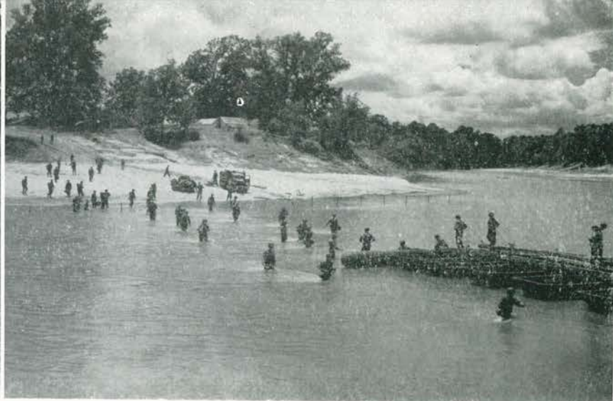
Louisiana maneuvers. 320th Engineers installing bridge across Sabine River that separates Louisiana and Texas
