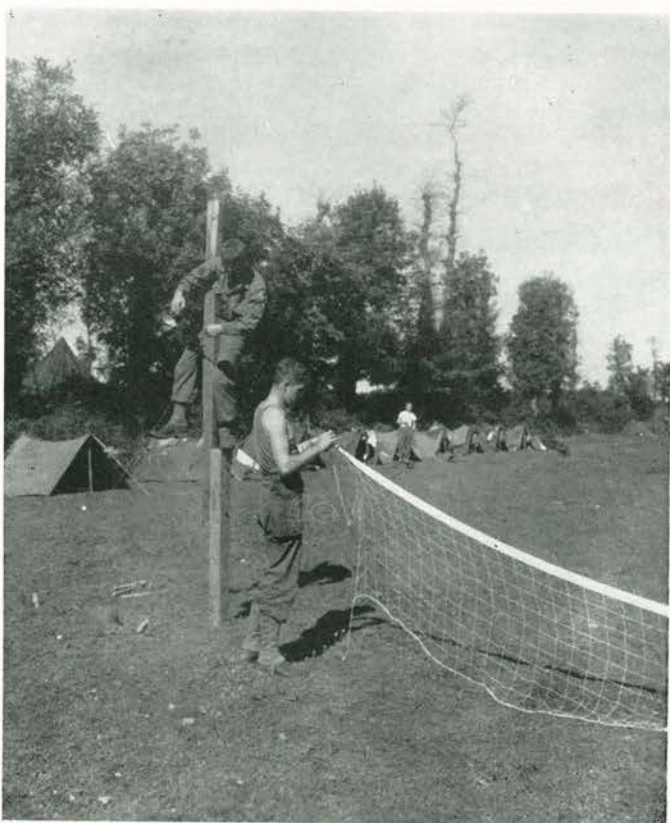
Trevieres, France. Bivouac area, Headquarters and Service Company, Sergeant Thomas and Sergeant Stoller erecting a volley ball net. September, 1944
