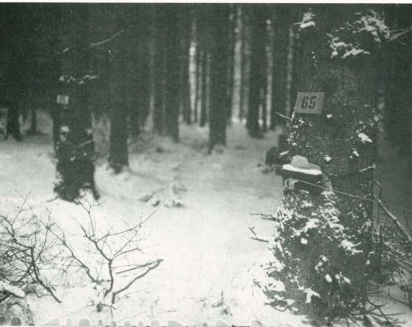
Close up of abatis showing how demolition is placed in tree prepared for demolition, as part of defense plan
