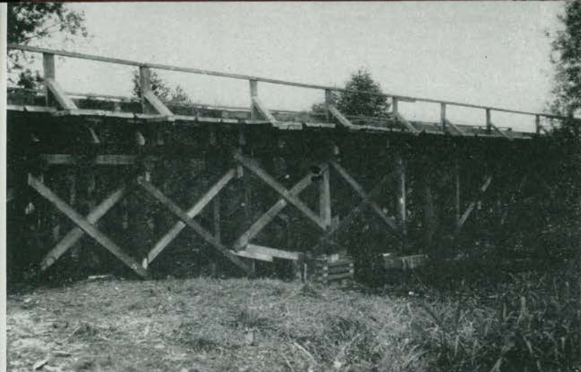
Timber trestle bridge constructed across small stream near Olfen, Germany
