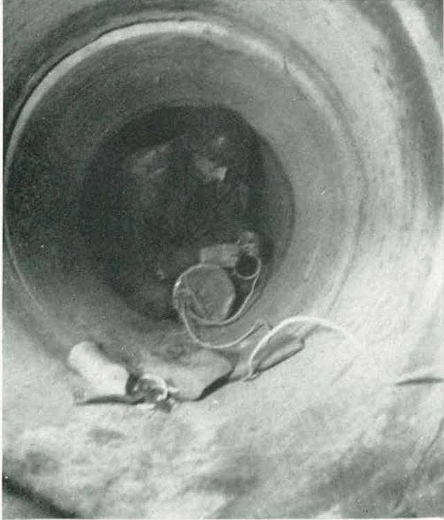
Wiring of culvert for demolition being prepared by Company C
