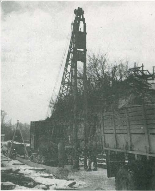
Adjusting pile driver in preparation of bridge site
