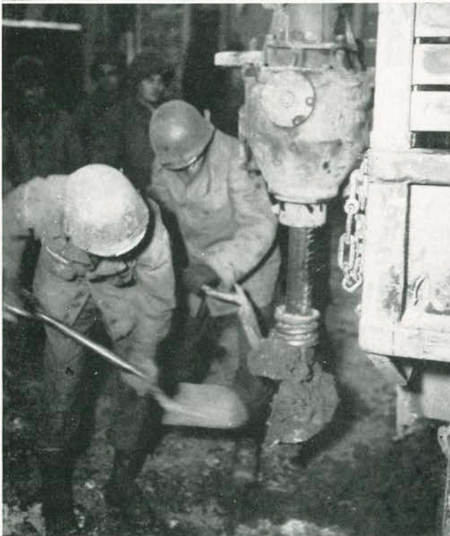
Private Jensen and Private First Class Carter of Company A cleaning blades of earth auger while preparing road crater in defense plan
