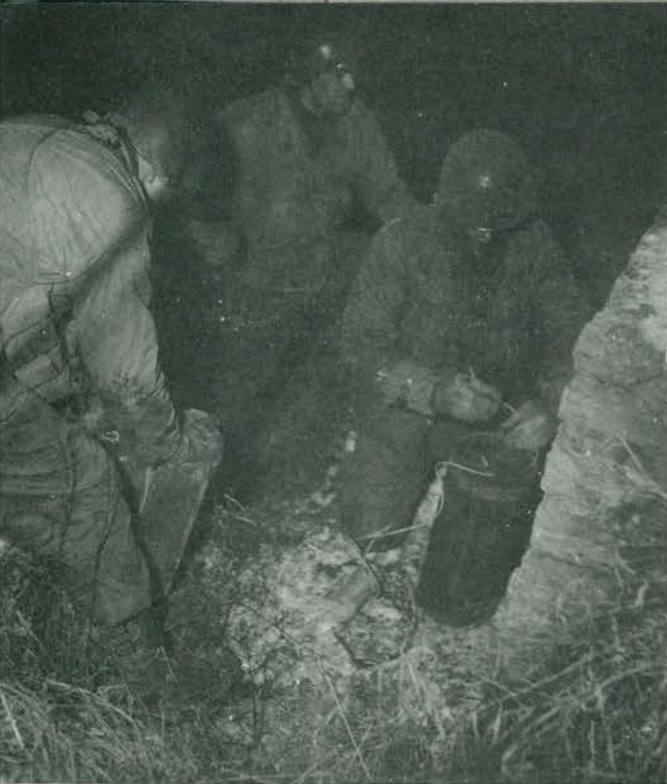
Company C men, with Sergeant Farrel in charge, attaching Primacord fuse to a cratering charge in preparing a culvert for demolition
