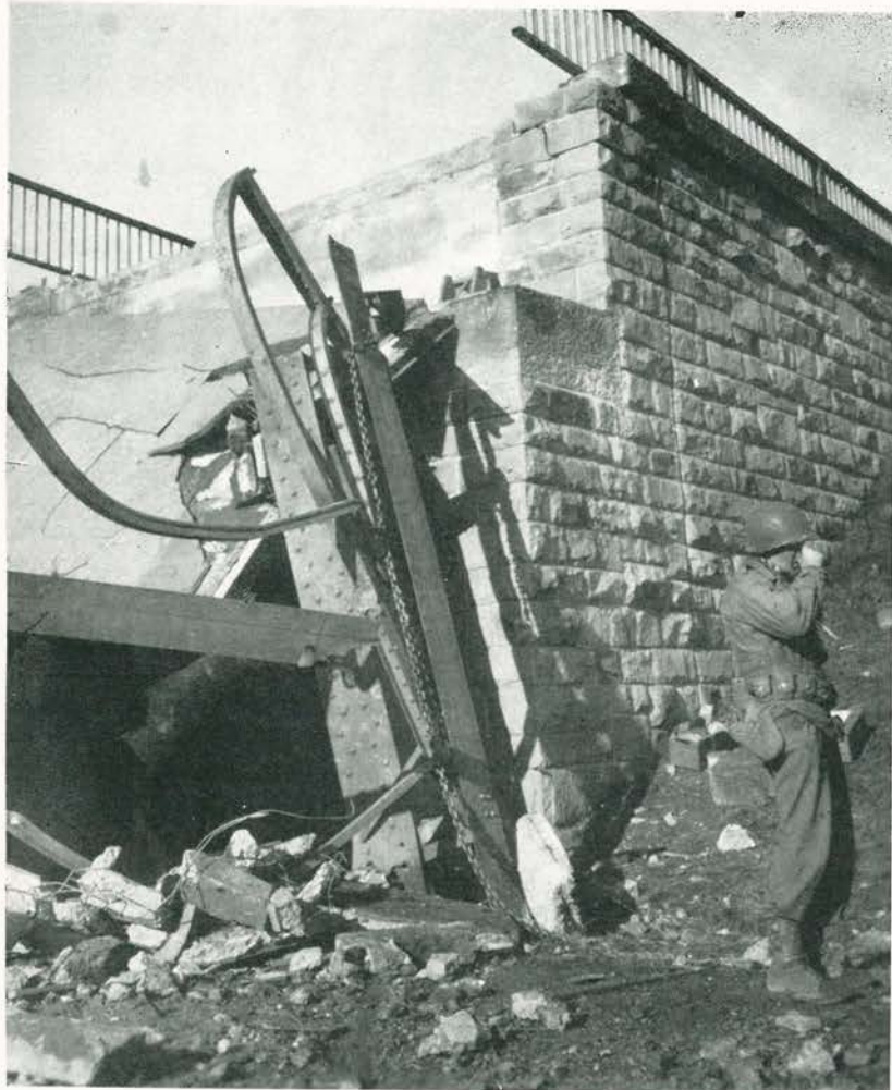
Close-up view of bridge dropped across autobahn. Note clean cut
