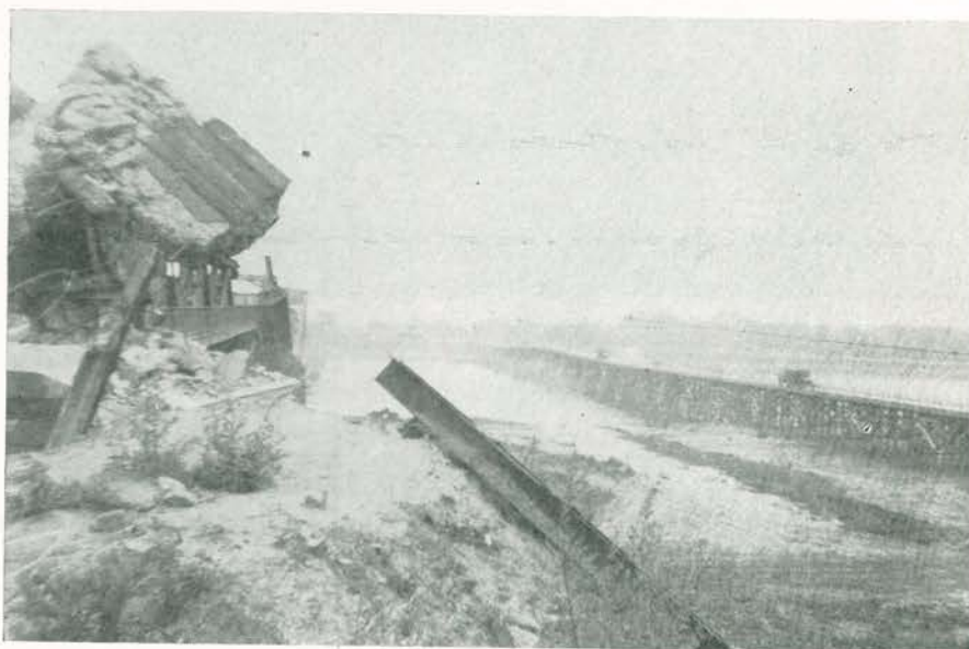
320th Engineers crossing Rhine River bridge, demolished on left
