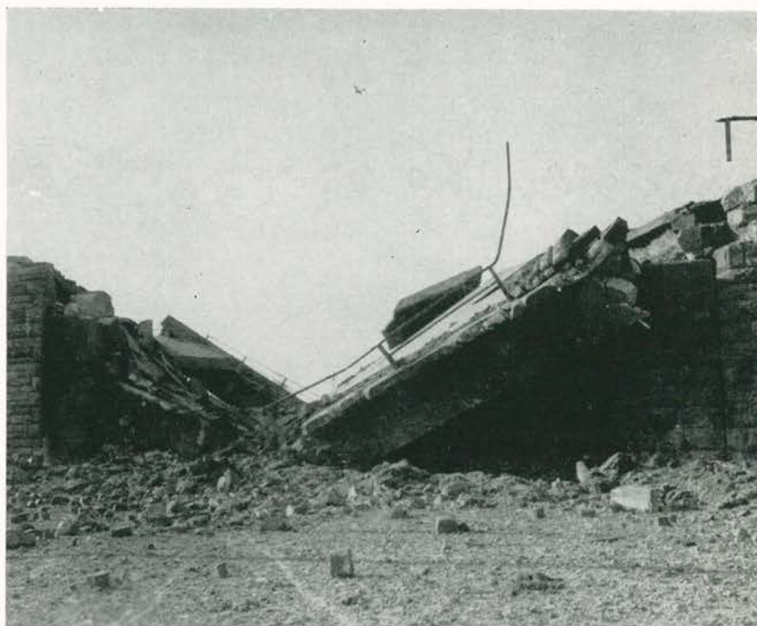
Bridges blown across autobahn by German troops in retreat
