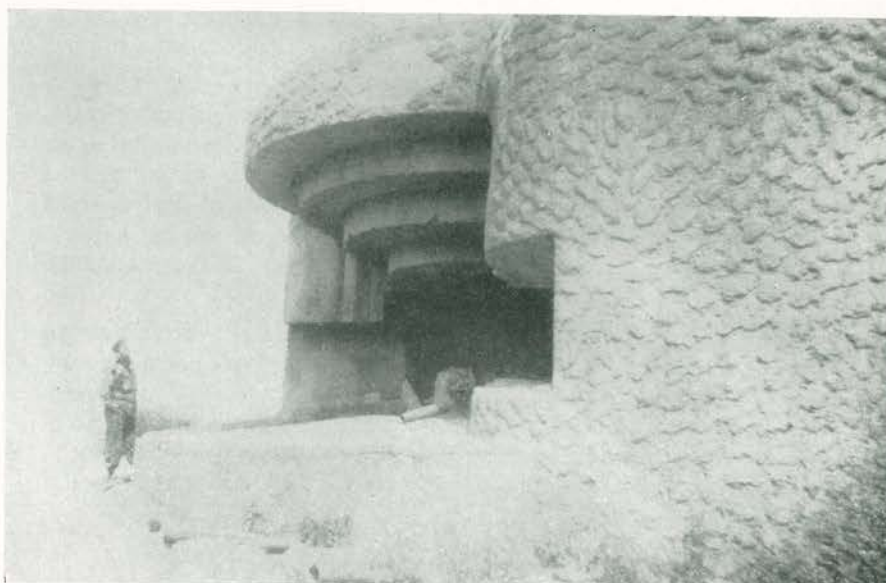
Fortification at Le Havre, France. This is typical of numerous installations that dotted the cliffs in vicinity of Le Havre
