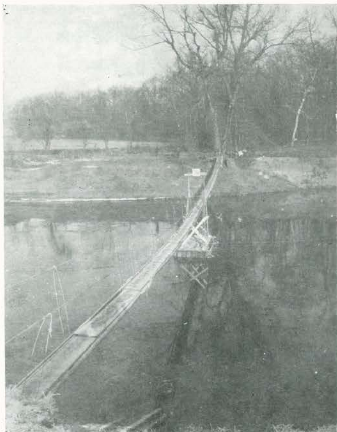
Suspension foot bridge with floating support built under Lieutenant Keough's supervision, Company C
