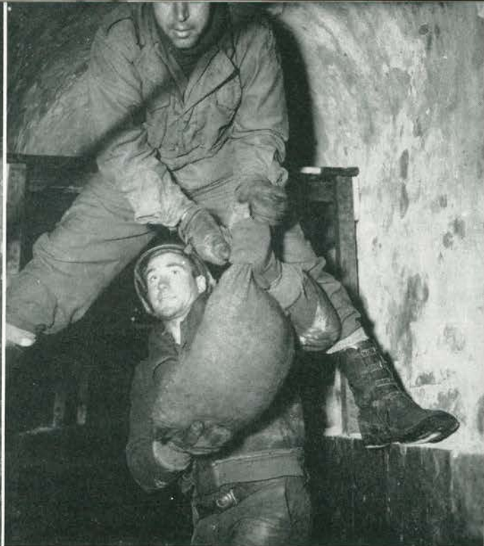
Further preparation for demolition culvert near Tromborn, France
