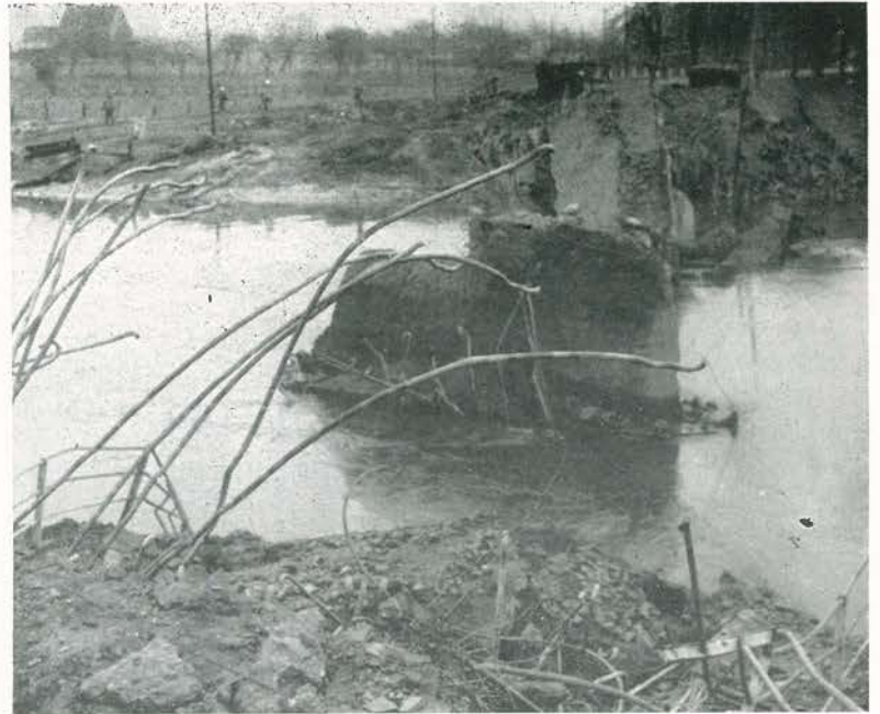
Bridge demolished across the Lippe River
