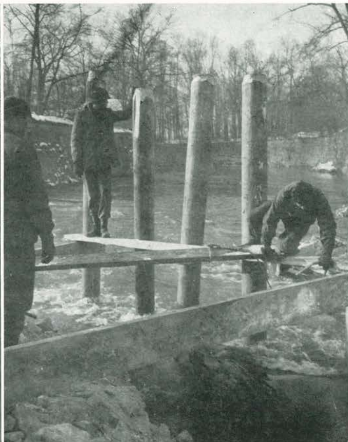
Placing planks into position at bridge site north of Saarlautern
