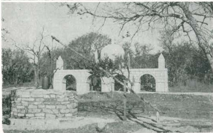
Finished spillway to dam constructed by 320th Engineers at Camp Swift, Texas. Close-up of structure in Branntown, Camp Bullis, Texas, 1943.
