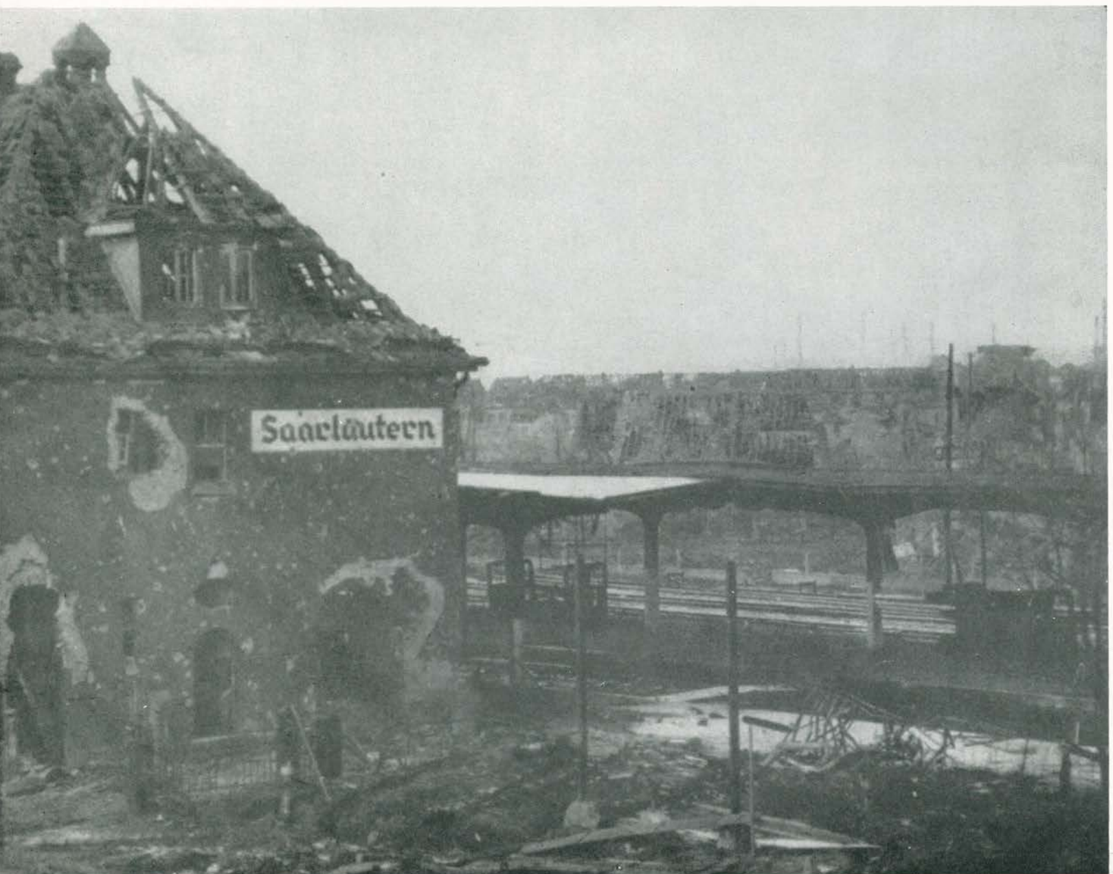
This is what was left of the Saarlautern railroad station when German artillery was through pounding the city
