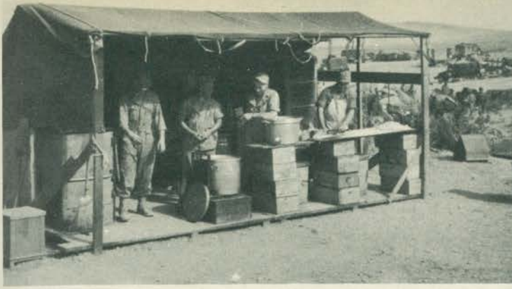
Kitchen on "Dust Hill"
