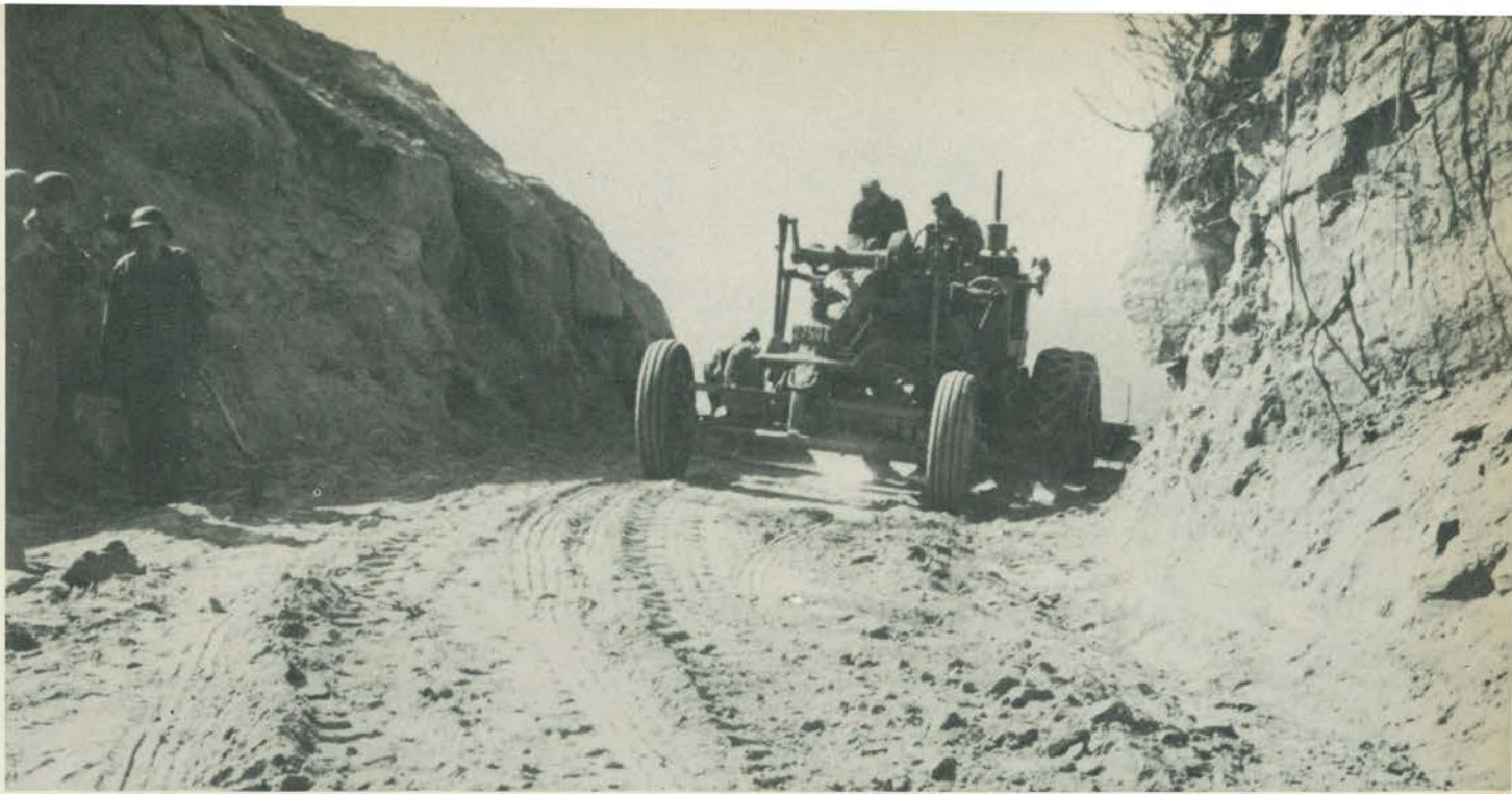
Above Riola: Road Building
