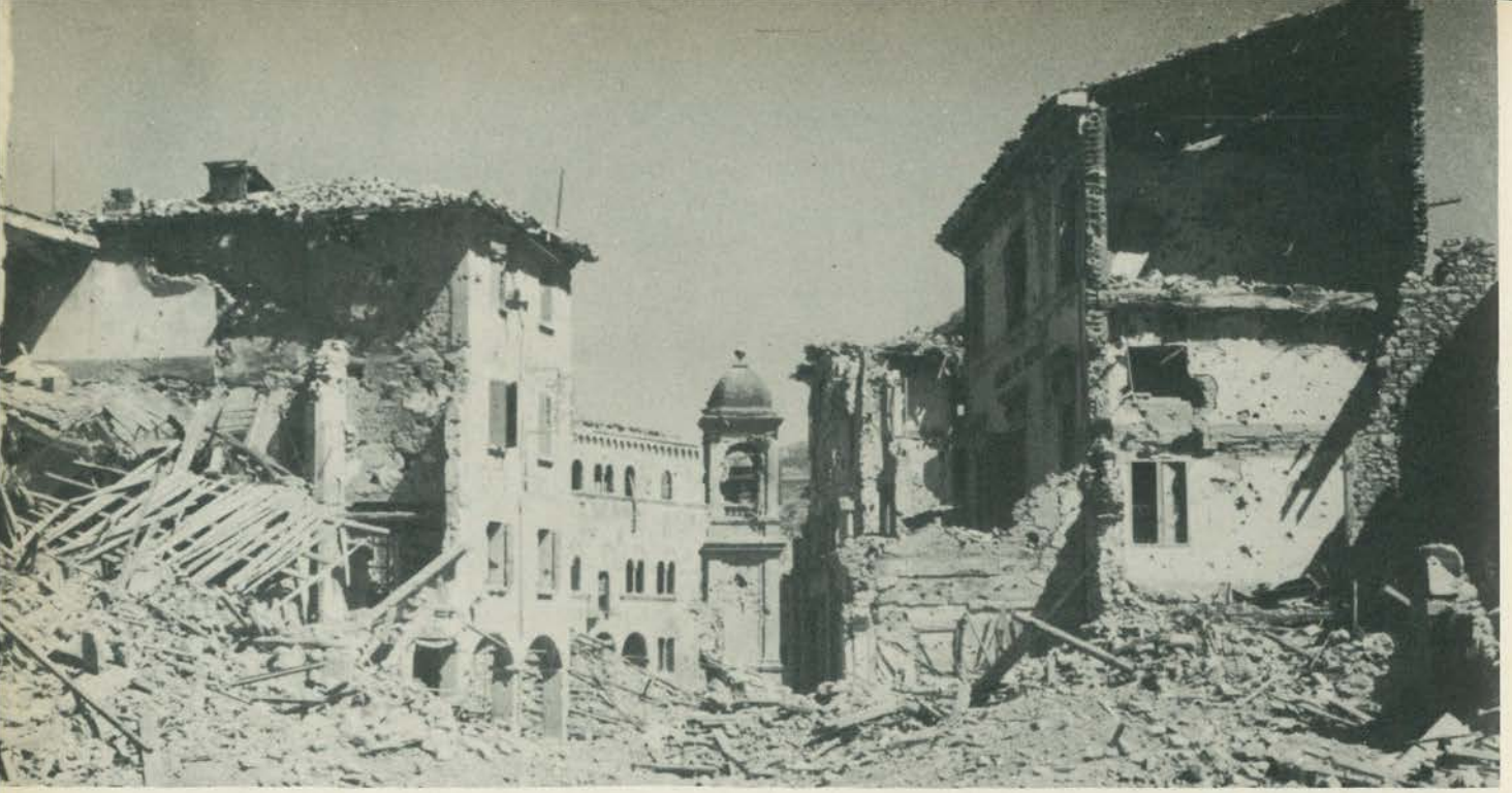
Vergato: Blocking the Road to Bologna
