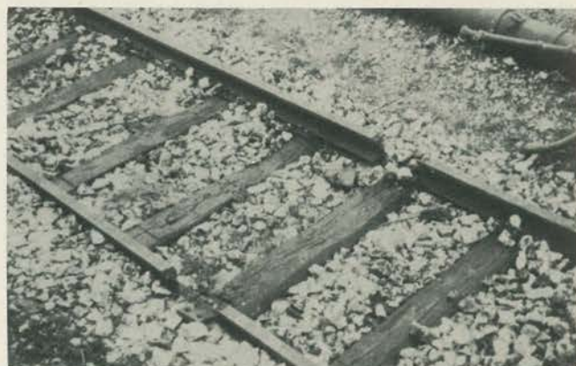
Near Rome: Railroad Demolition
