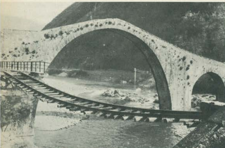
Pte. d. Maddalena: Railroad Demolition
