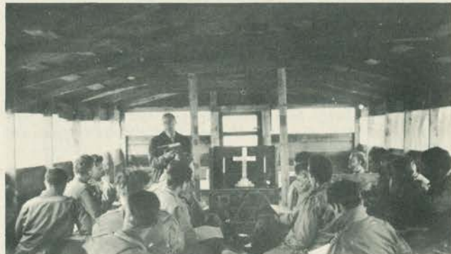
Service at Battery A
