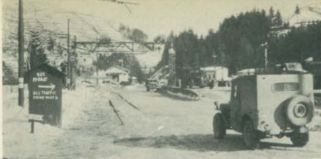
Pracchia: By Pass
