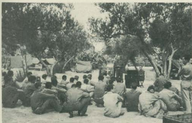
Service at Battery C
