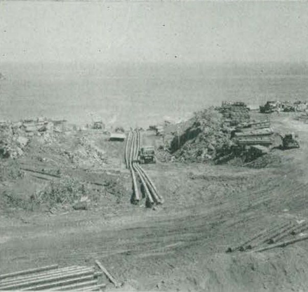
A great system of 90th-built pipelines, connecting with tankers-fed submarine pipelines, supplies the huge gasoline tank farm on Iwo. The system includes fueling loops from the tanks to the hard stands along the airstrips where planes are fueled. In addition to construction, 90th men maintained and operated the fueling loops and pipelines for many weeks after the
