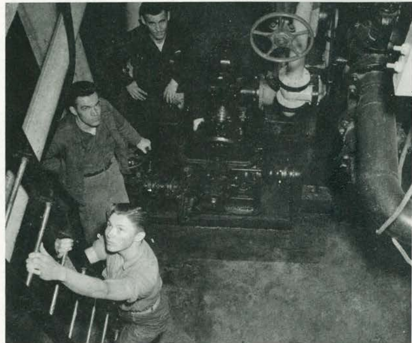
Fuel Oil Maintenance Crew and Equipment
