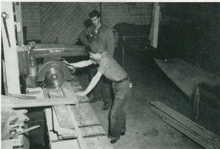
Interior of Carpenter Shop
