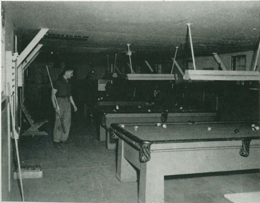
Top: Library and Recreation Building Bottom: Pool-Room — Recreation Building
