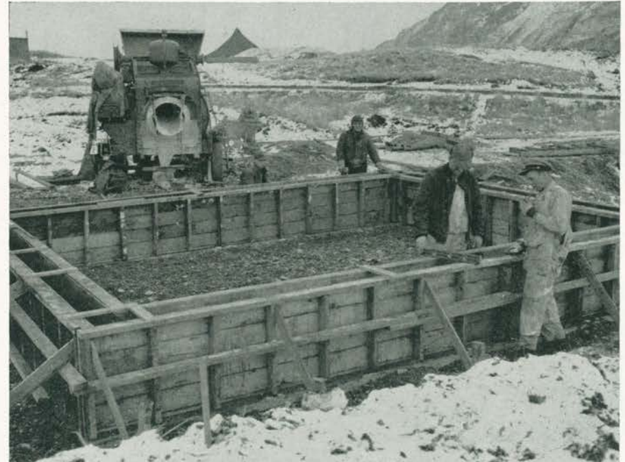
Generator Building Foundation Forms Set and Ready to Pour
