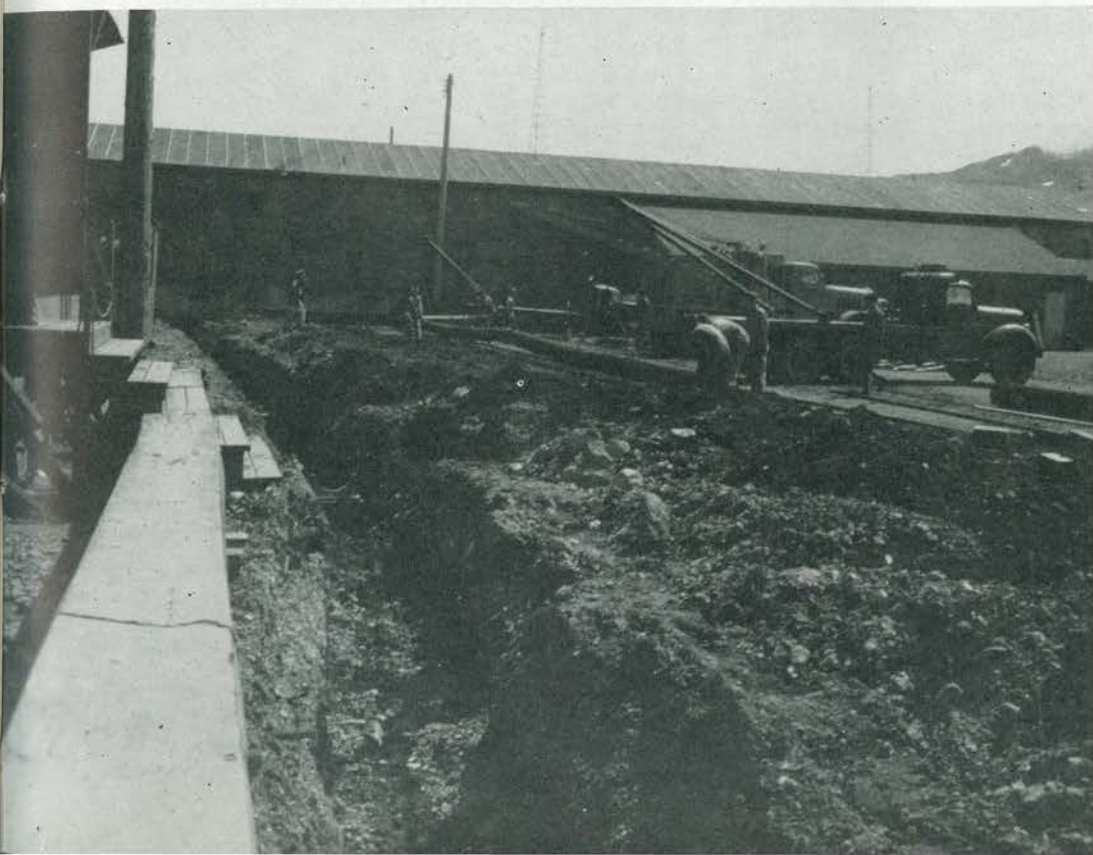
Placing Steam Line
