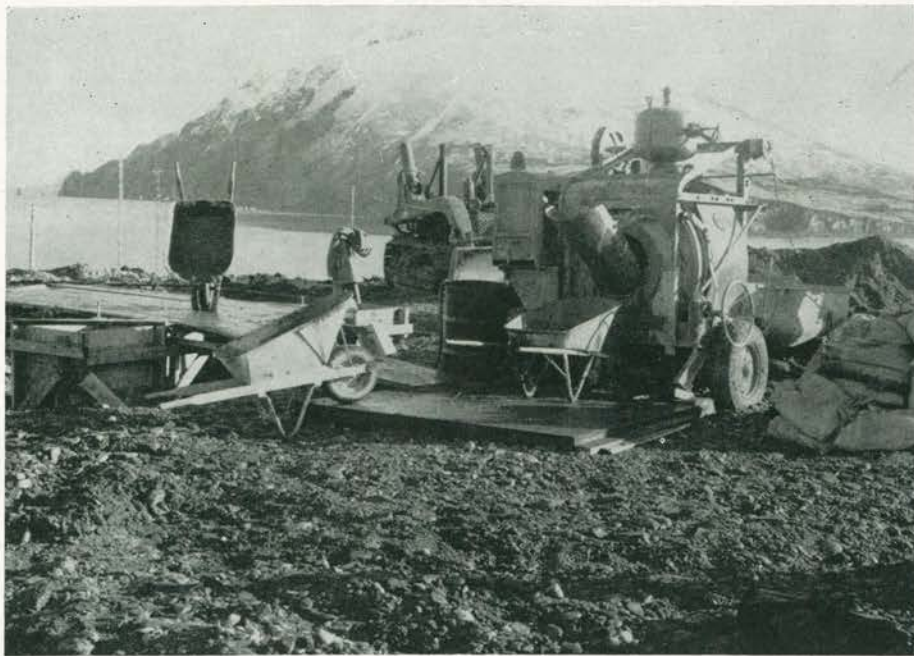
Pouring Foundation for East Tower
