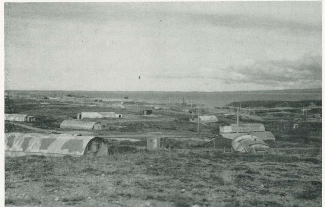
Quonset Huts Had to Be Half Buried to Withstand the Hundred Knot Winds
