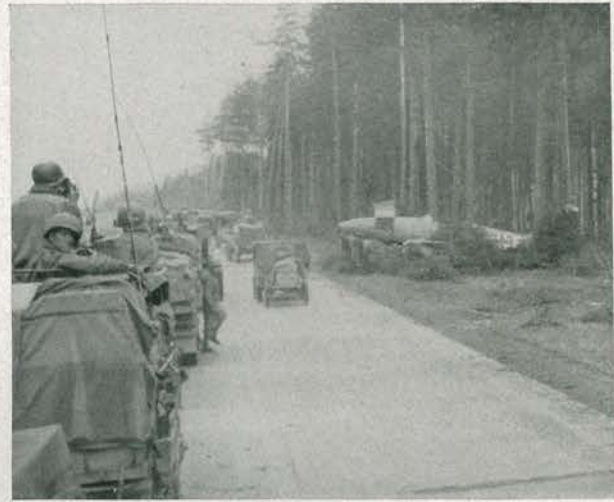
Battery column along the autobahn and a "jet"
