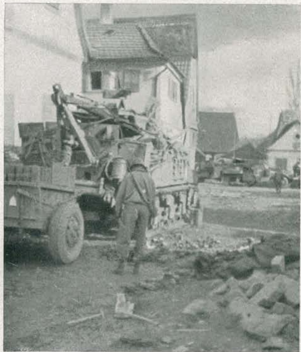
Motor maintenance worked day and night.
