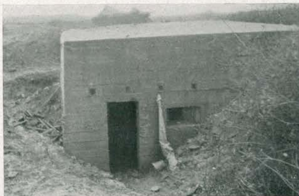
Our shell-shelter at Singling — A typical Maginot pill-box.
