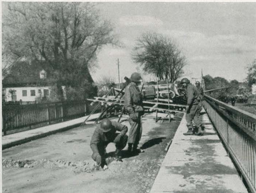
Engineers clearing planted demolitions from blockaded bridge in path of our column.
