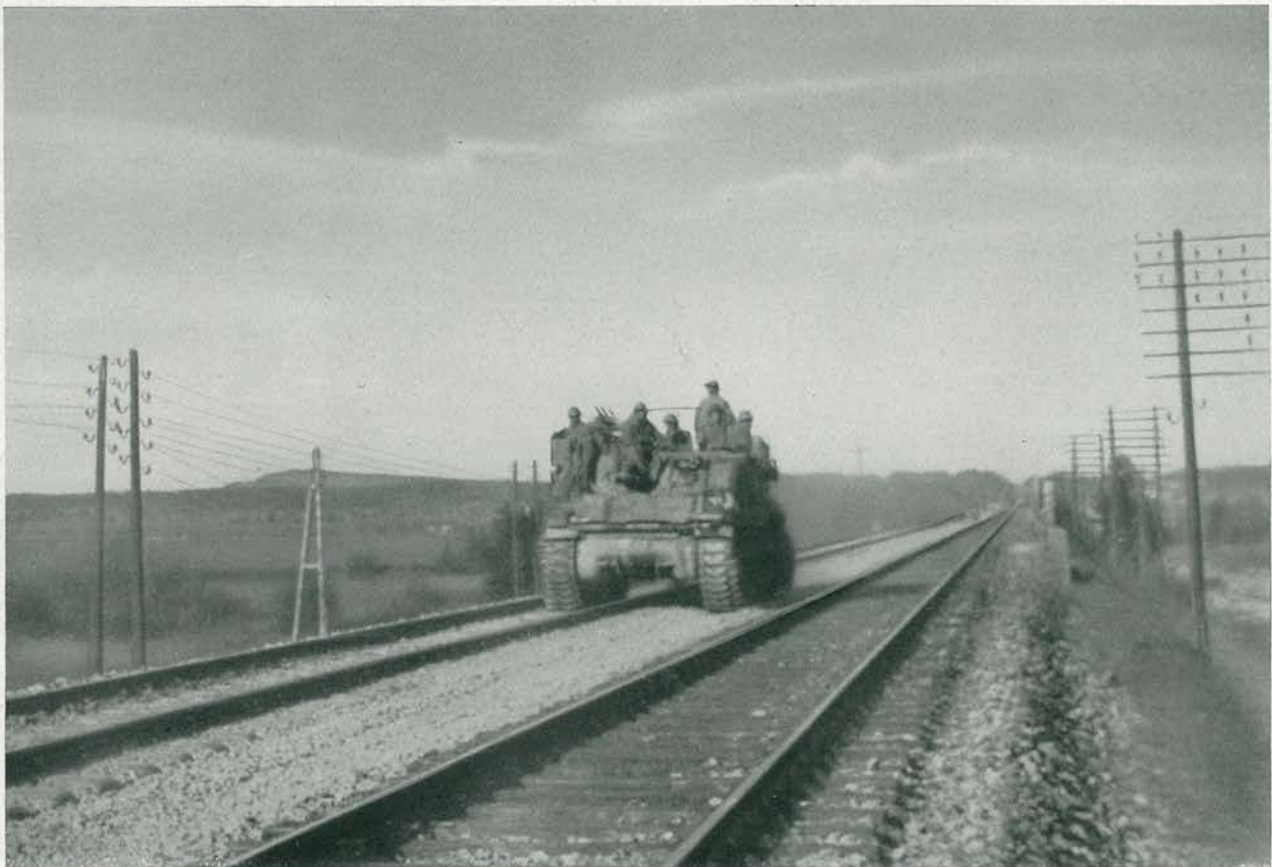
An M-7 takes the railroad bridge across the Lech River near Landsberg, Germany, as did the rest of the Bn that day.
