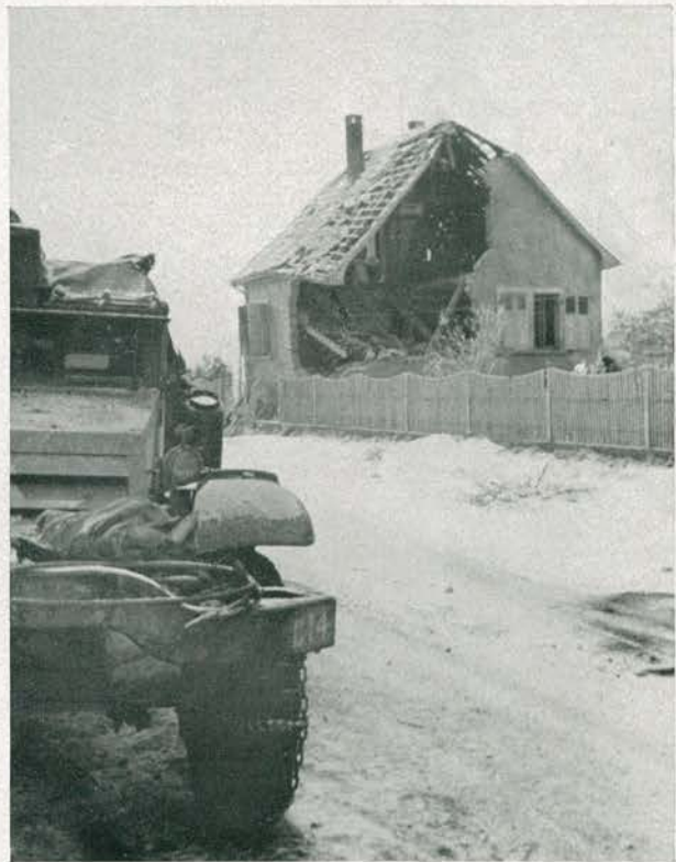
House that was hit twice at Bischwiller — just across the road from the "Exec".
