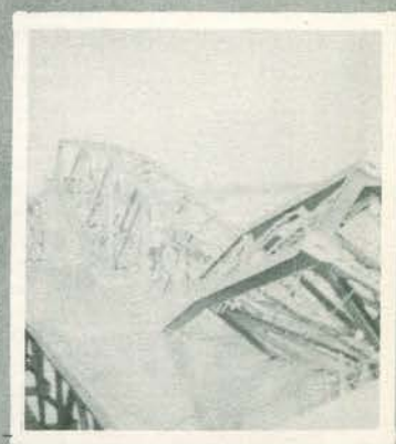
DEMOLISHED BRIDGE ACROSS RHINE RIVER—MAINZ, GERMANY
