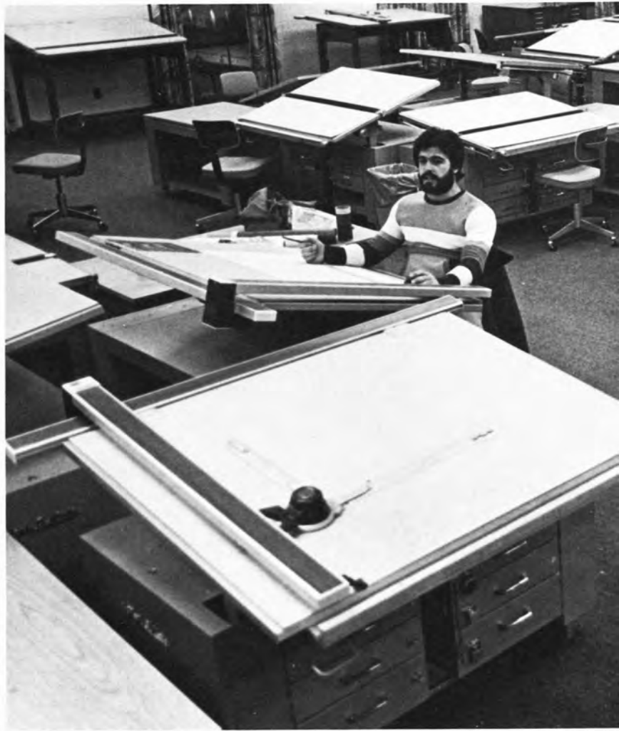
Greco drafting construction plans.
