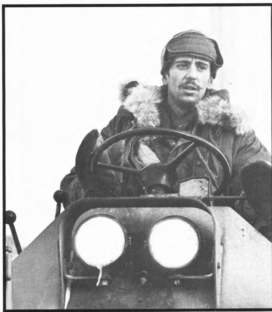
Army engineers from Fort Bragg, N.C. helped dig out the city.
