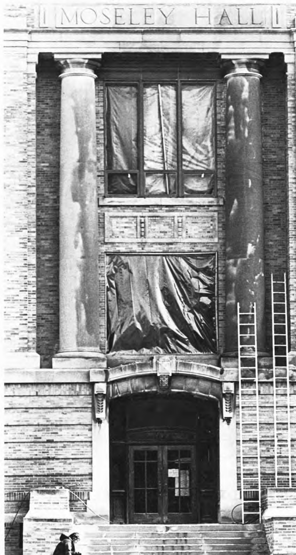
Moseley Hall renovation caused a classroom shortage.
