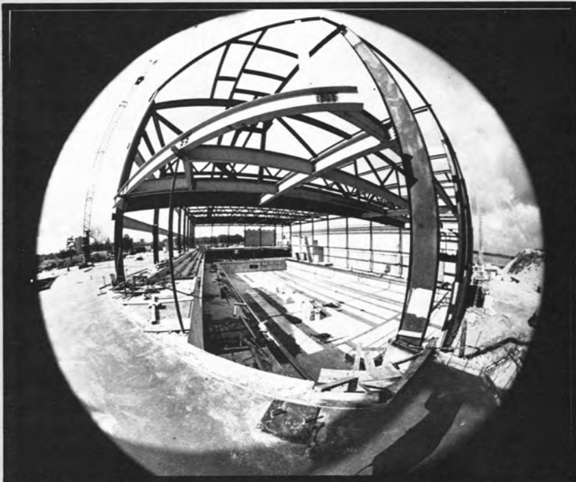
The Recreation Building takes shape.
