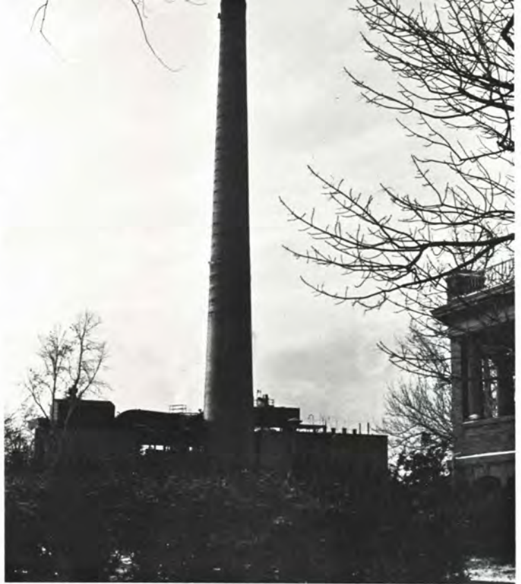
Coal is burned at the physical plant located on Thurstin Street to heat University dormitories. The plant's smokestack serves as a directional landmark for people who may not know their way around campus.
