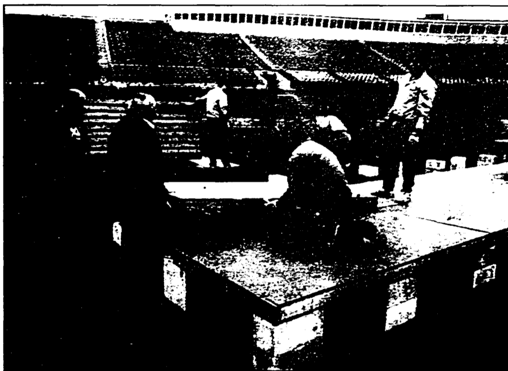
Crews from the physical plant build a platform for last Saturday's commencement.
