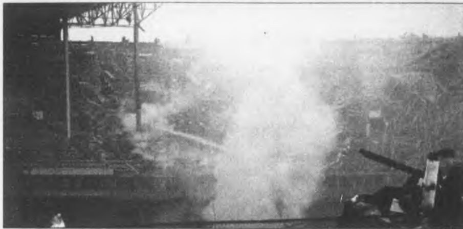
Adding insult to injury, part of Cleveland Municipal Stadium caught on fire Tuesday afternoon as welding sparks ignited roofing material behind home plate. AP Photo
