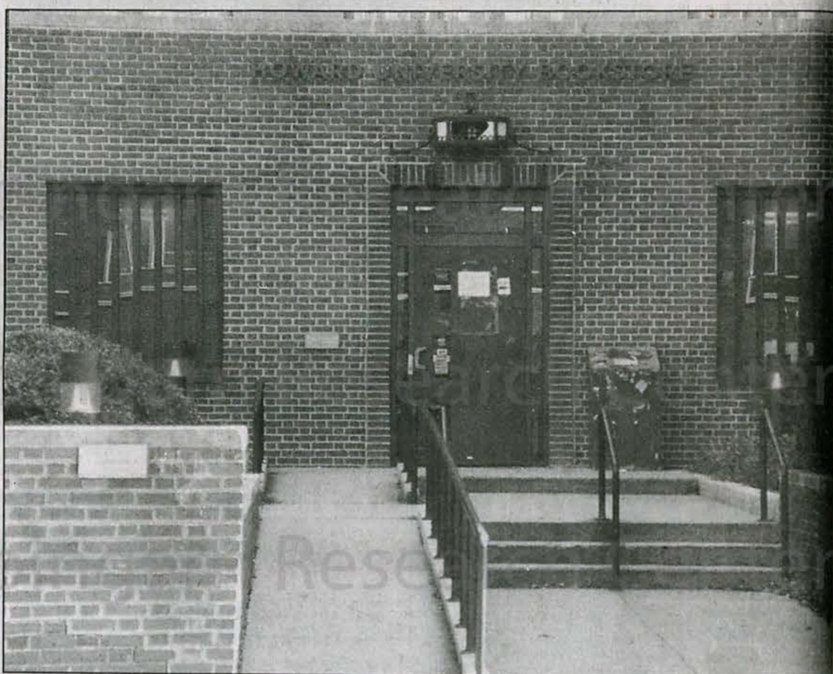
The campus bookstore needs to be recarpeted after flooding over Homecoming weekend.
