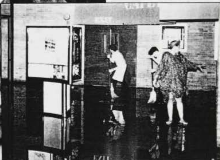
Director of Blackburn, Ms. Roberta McLeod orders clean-up as gallons of water flood the ground floor of Blackburn.
