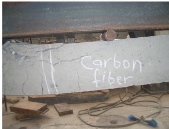
Figure 5: Failure mode of beam retrofitted with CFRP plates
