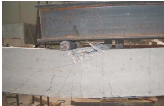
Figure 7: Failure mode of beam retrofitted with HSGS plates
