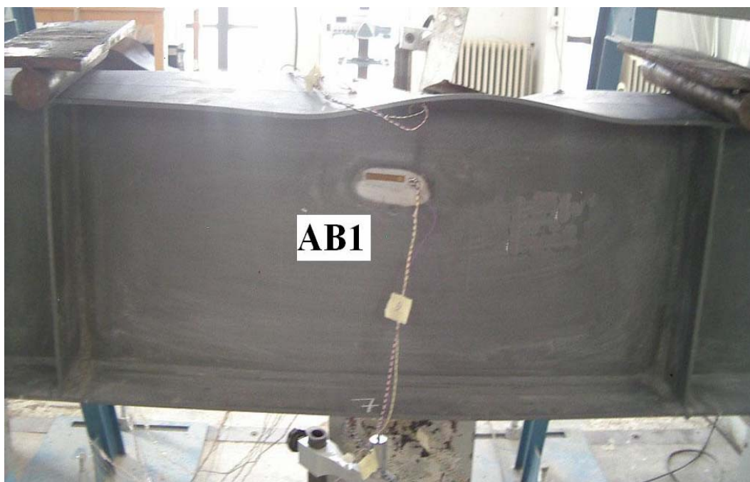
Figure (10): Local Buckling Mode in Beam AB1.
