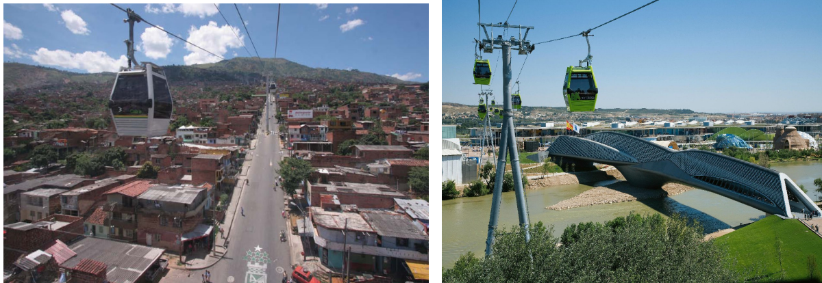
Figure 2: Cable cars in Medellin, Colombia ( left ) (Source: www.myclimate.org/carbon-offset-projects ) and Saragossa, Spain ( right ) (Photo: Leitner)
