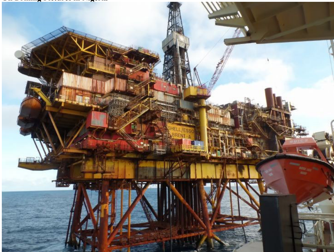
Oil Rig Photos. No: 3109 Contributor: Phillip Roncone Year: 30 th January 2017
