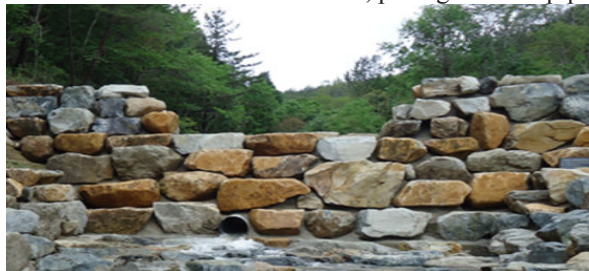
Figure 2. A check dam with structural improvement to enhance drainage
