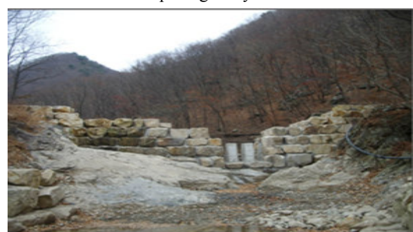
Figure 7. Structurally improved check dam showing visible passage ways from upstream to downstream. Water pollution is mitigated as water easily flows and carries materials along.
