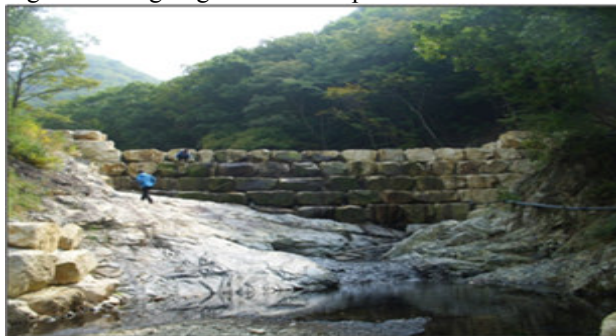
Figure 7. Structurally improved check dam showing visible passage ways from upstream to downstream. Water pollution is mitigated as water easily flows and carries materials along.
