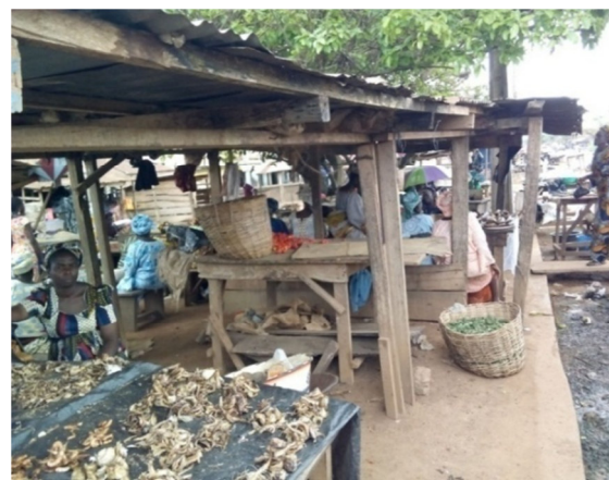
Plate 8: Showing Temporary structure at Ise/ Orun Market
