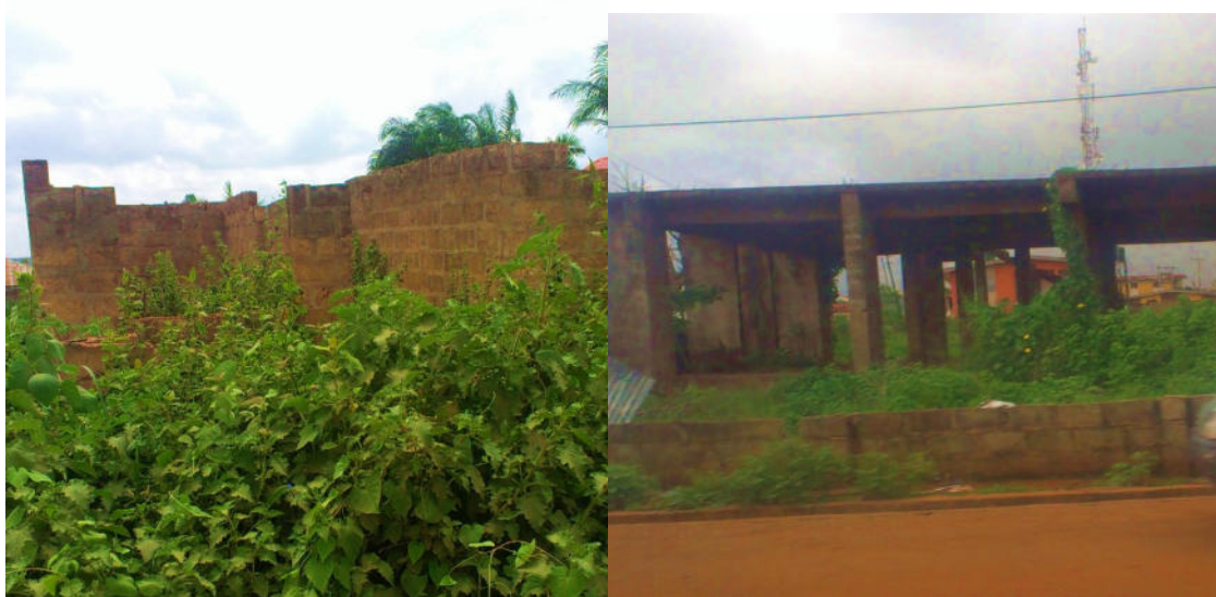
Plate 3: Uncompleted and Bushy Abandoned Structures in Maraba Area. Source: Author's Field Survey, 2015
