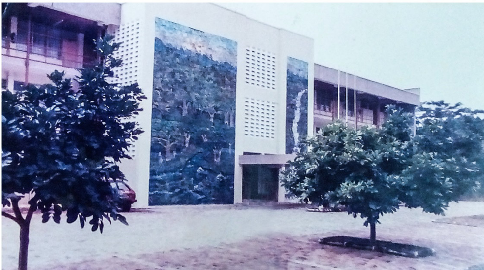
Figure 11. Ceramic mural mounted on the administration block of Forest Research Institute of Ghana at Fomesua
