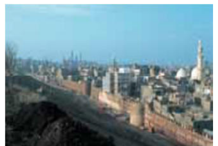
Figure (9) Ayyubid wall Restoration
