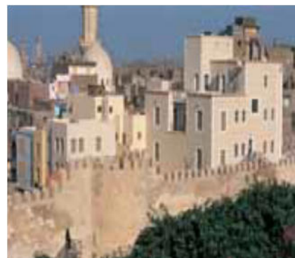
Figure 12. Housing rehabilitation in Darab Alahmar Neighborhood
