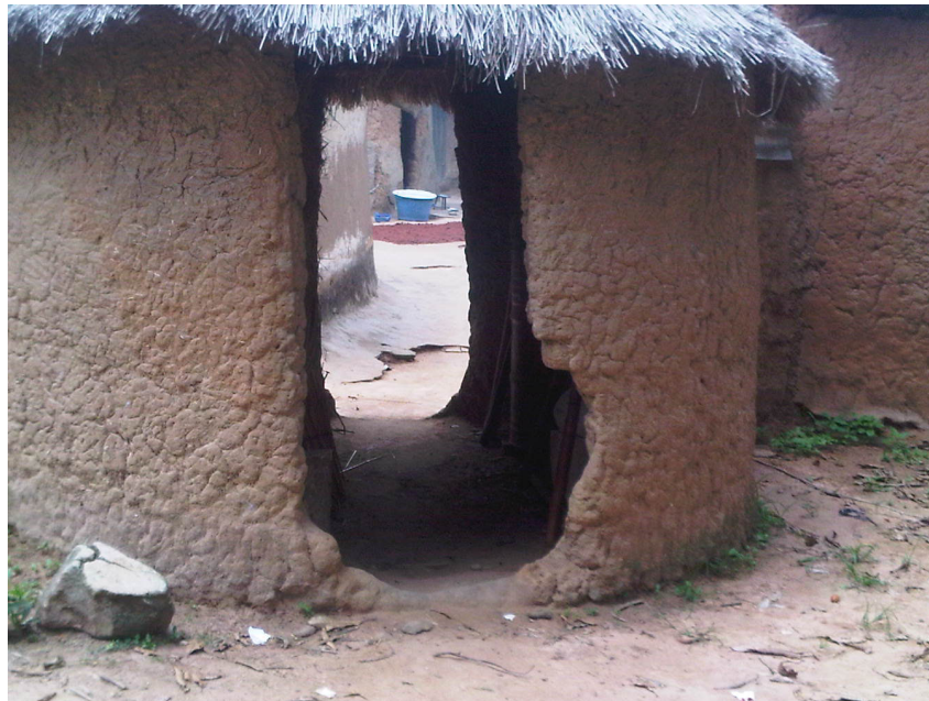
Plate 8: Mud used for building up walls Author's fieldwork.2011
